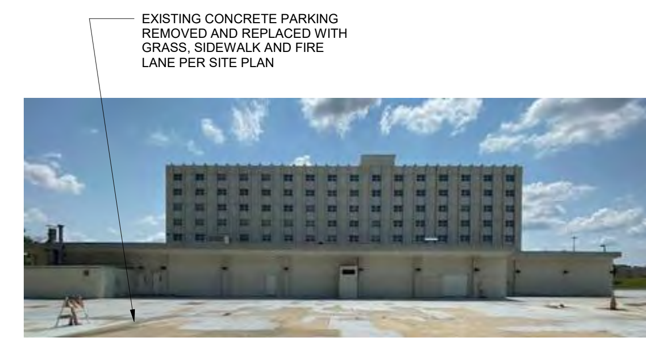
NORTH ELEVATION - EXISTING
