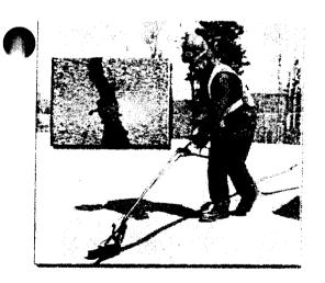
CRF® Restorative Seal is a petroleum oil and water cationic emulsion. Unlike standard asphalt emulsion, CRF® does not harden or "dry out" Designed as a one component emulsion that effectively repairs cracks in concentrated form, CRF® provides a excellent pavement restorative seal when applied in diluted form.
