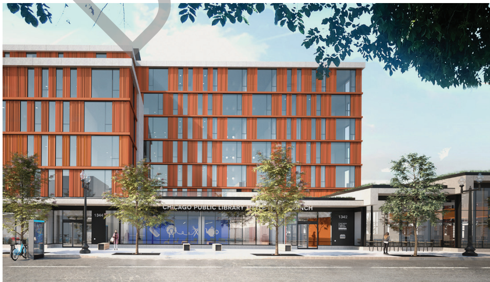
Photo credit: SOM • The Roosevelt/Taylor library combines LIHTC, CHA and market rate units in the Little Italy community on the Near West side with the modernized version of the Little Italy branch of the Chicago Public Library designed with activity space for community and residents.
