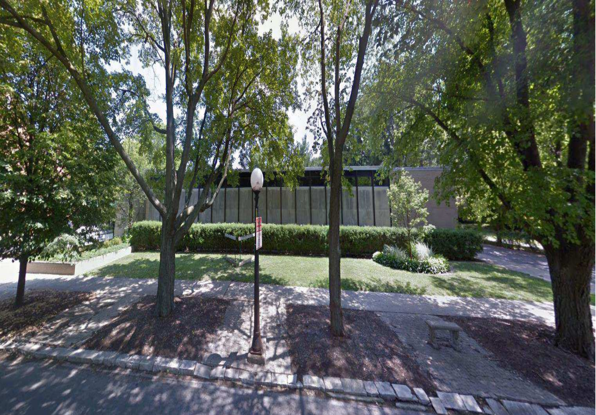
North Facade and North West Corner facing Moss Ave
