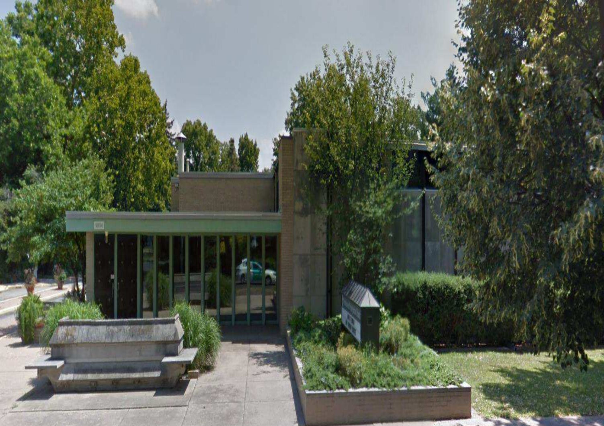
North East Corner facing Moss Ave
