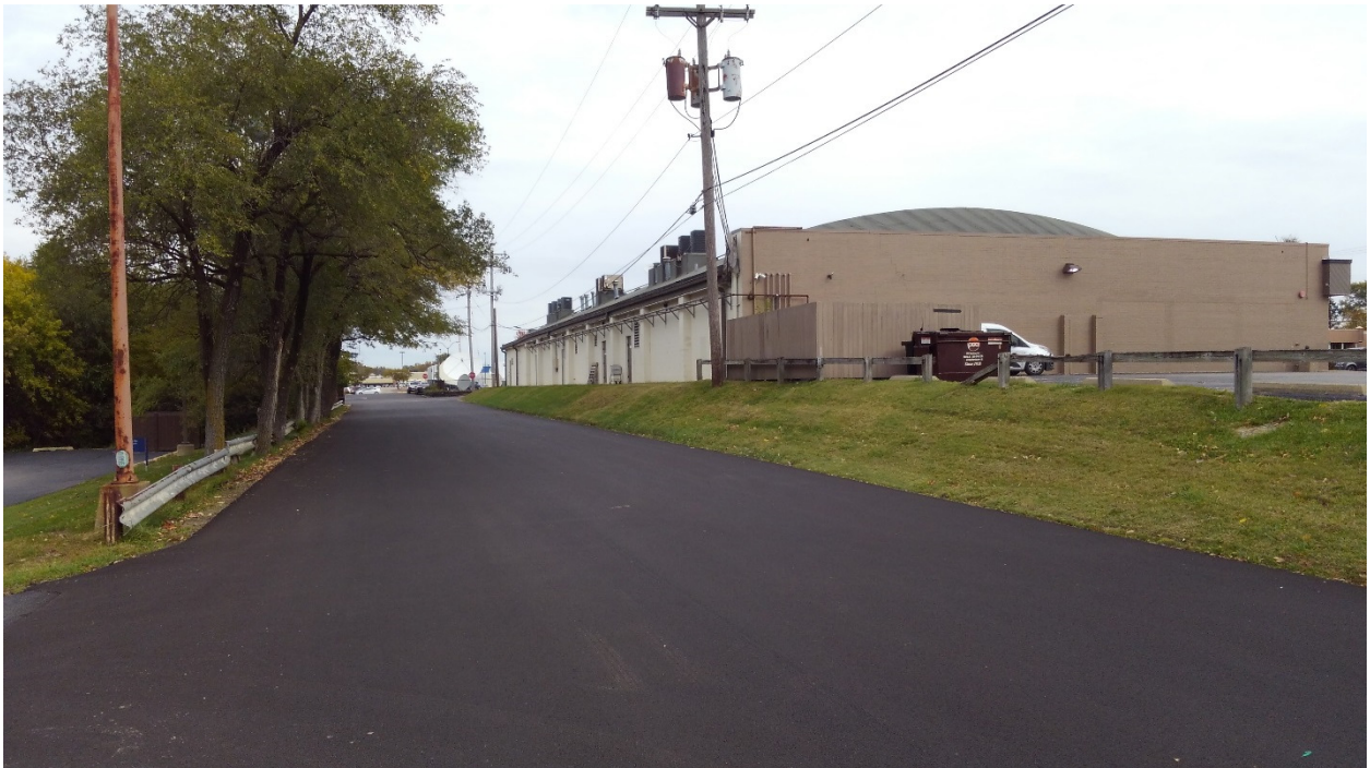
Looking North at South and West Sides of Building
