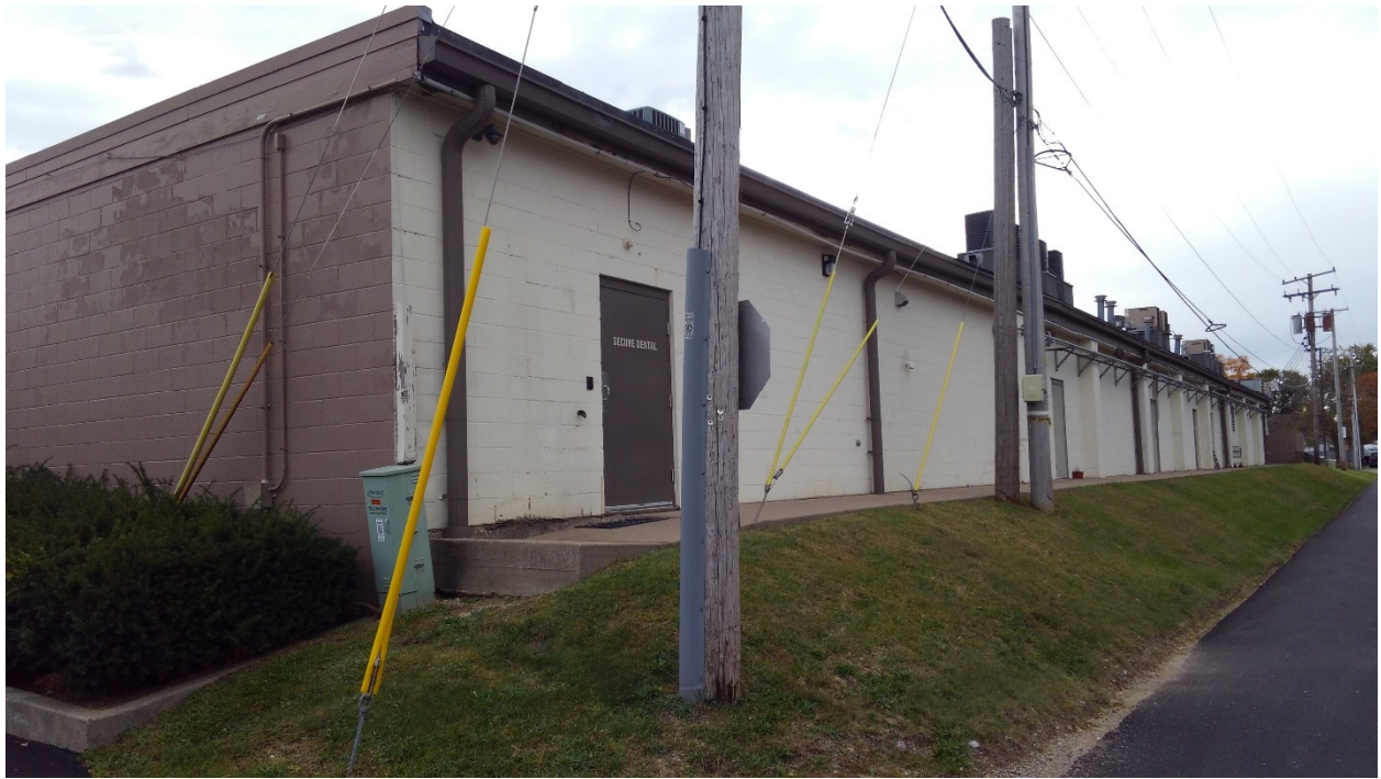
Looking Southeast at West Side of Building
