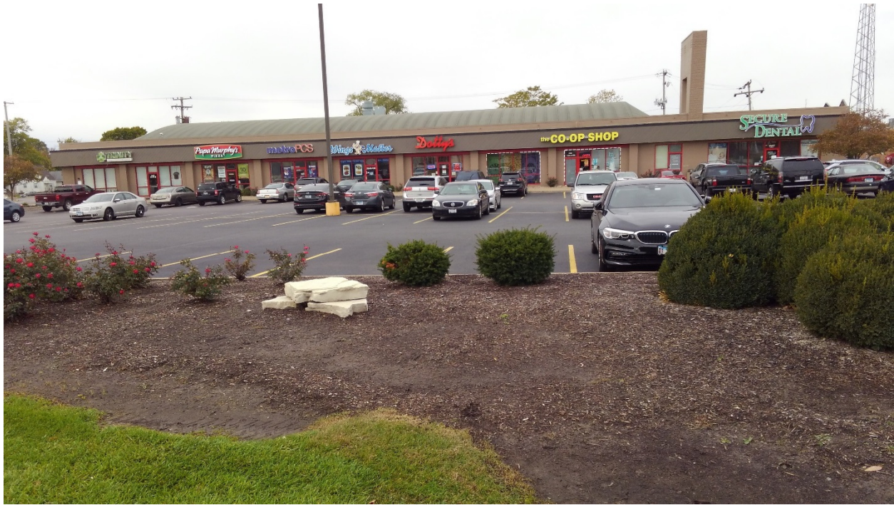
Looking West at East Side of Building
