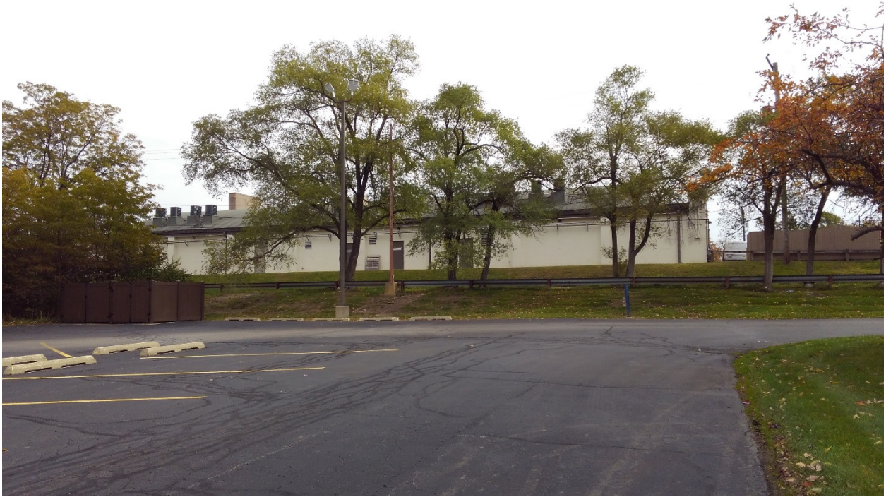
Looking East at West Side of Building
