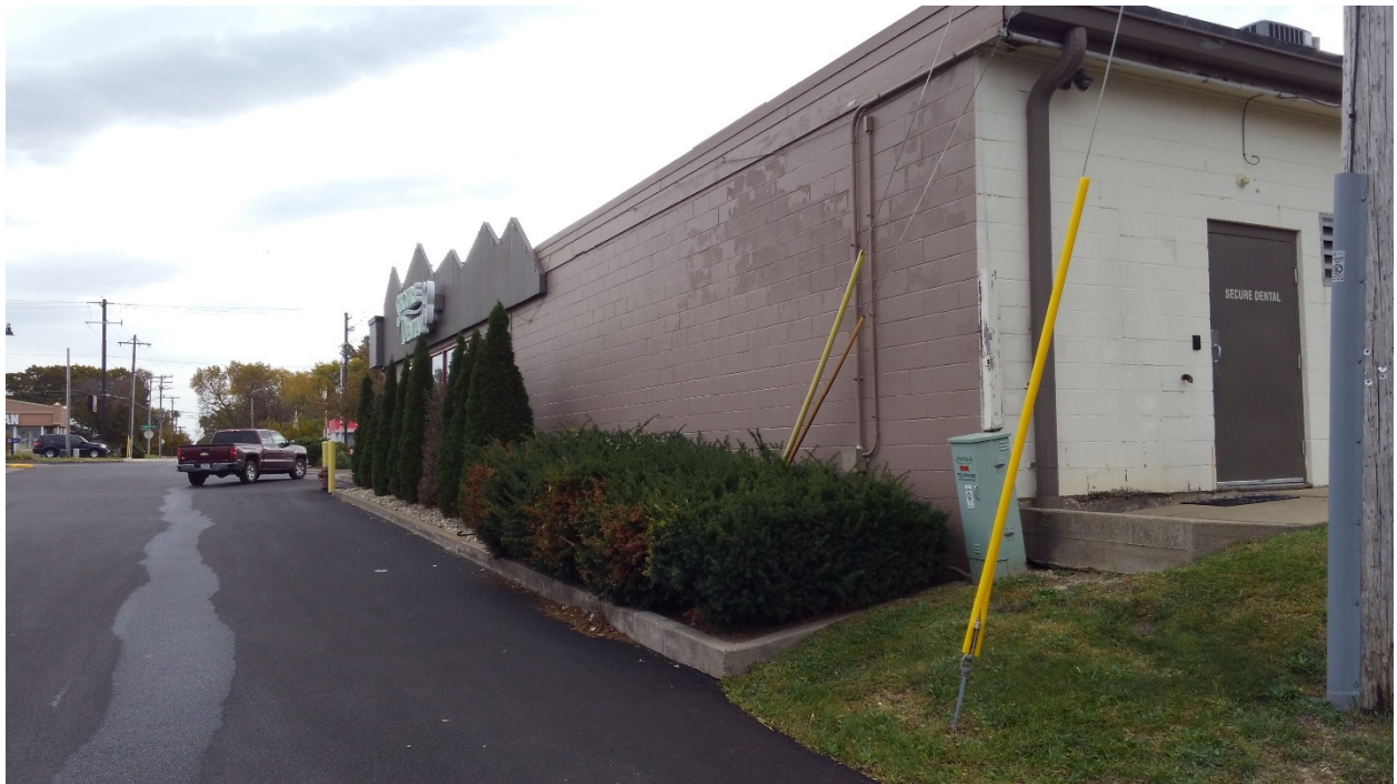
Looking East along North Side of Building
