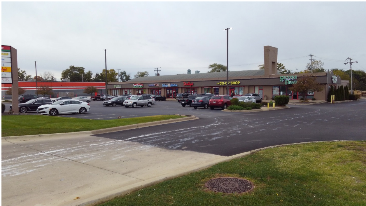
Looking Southwest at East Side of Building
