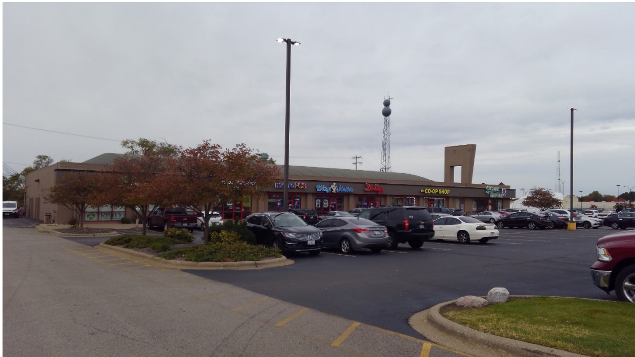
Looking Northwest at East Side of Building
