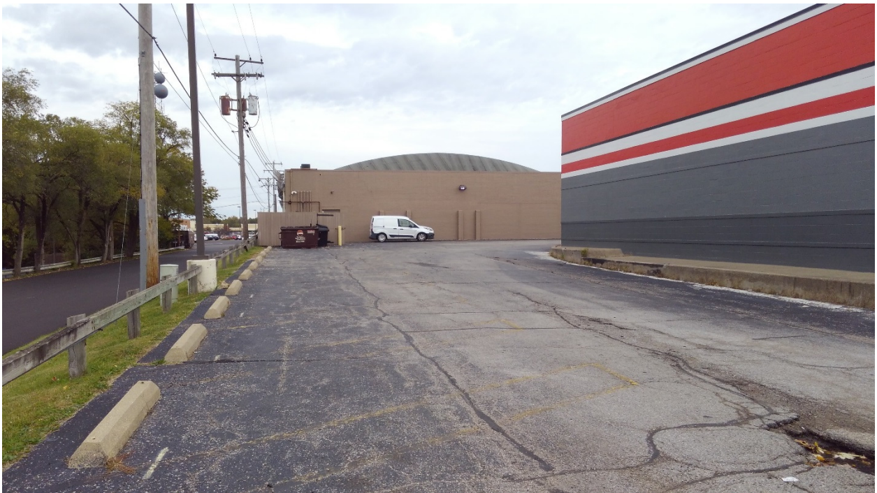
Looking North at South Side of Building
