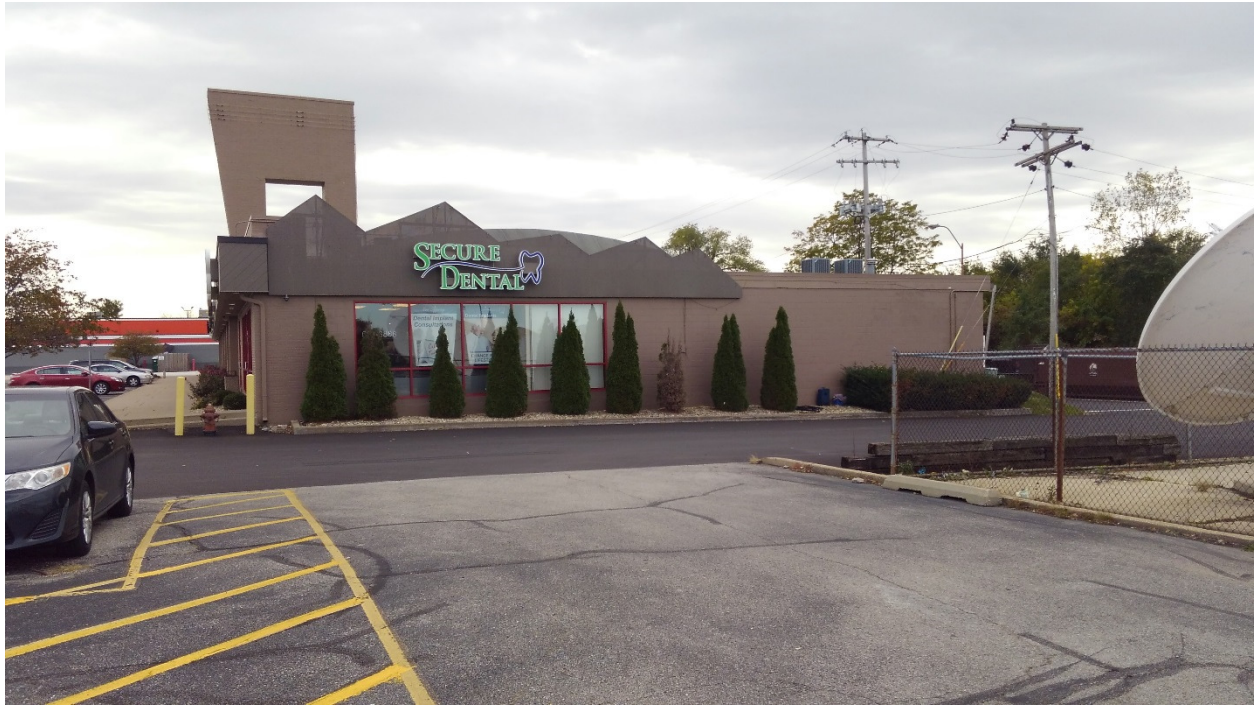
Looking South at North Side of Building
