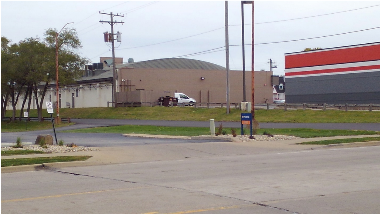
Looking Northeast at South Side of Building
