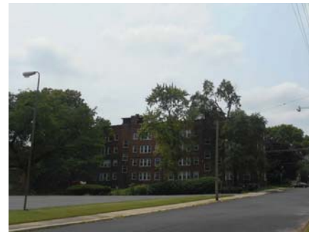
4 EXISTING EAST VIEW OF BUILDING SCALE: N.T.S.
