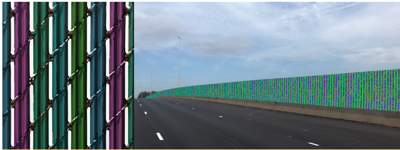
Colored Polycarbonate Insert Through Chain Link
