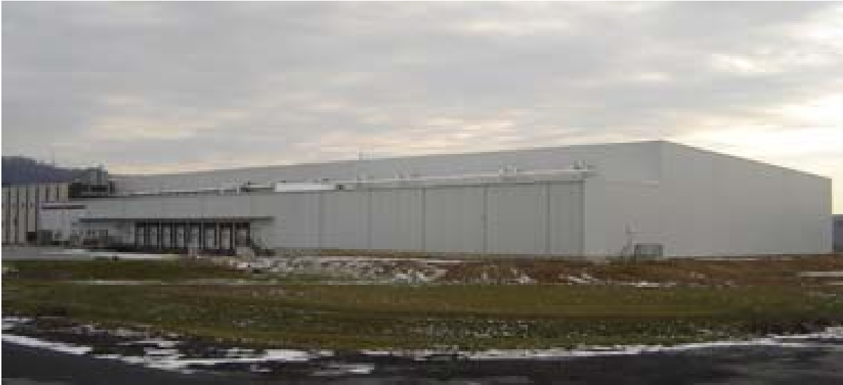
Freezer / Cooler Building for Kencor Ethnic Foods, Inc.
