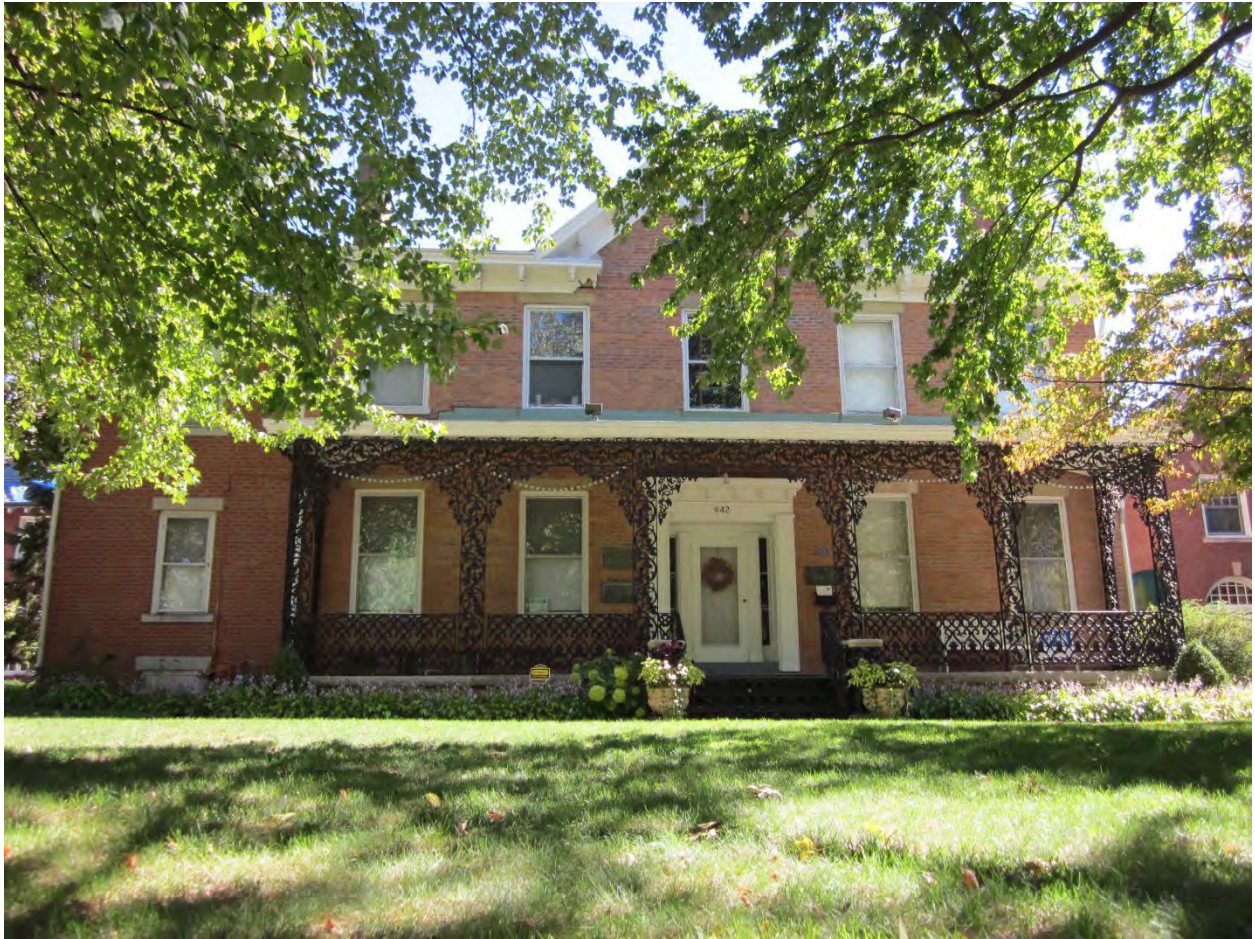
Photo D • Current view of Glen Oak Ave façade (current front façade) of Flanagan House
