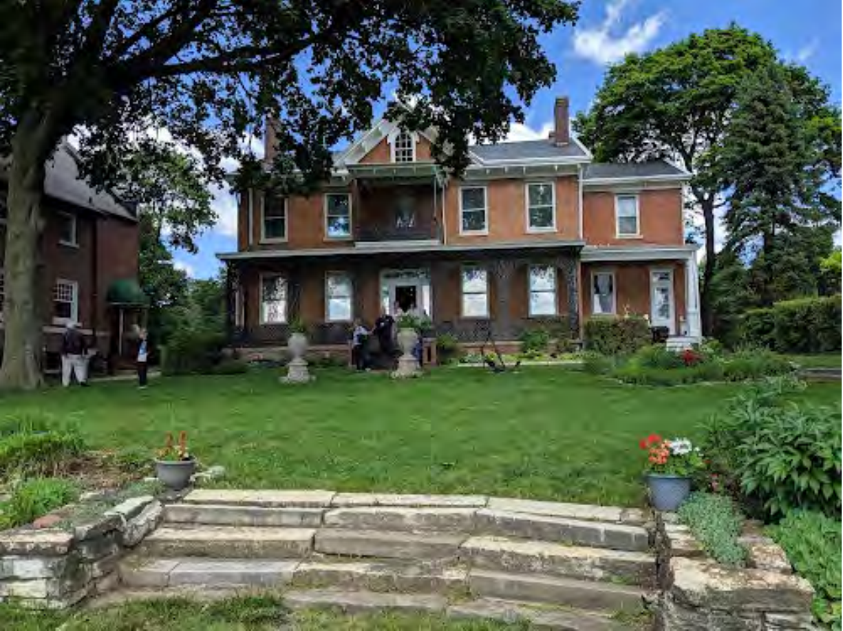
Photo C • Current view of bluff façade (former front façade) of Flanagan House
