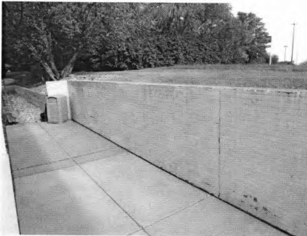
47. Retaining wall along south elevation
