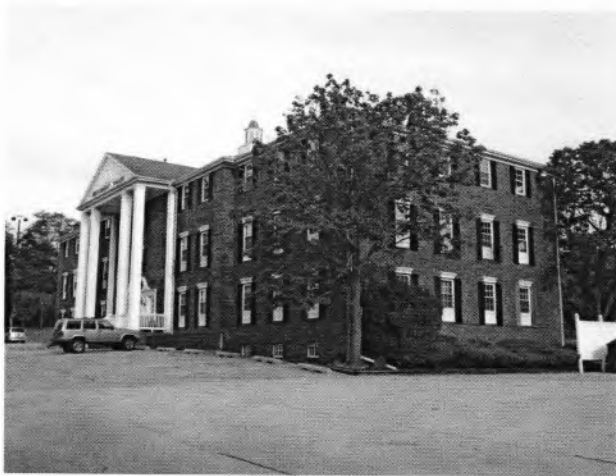
3. Northwest corner of building
