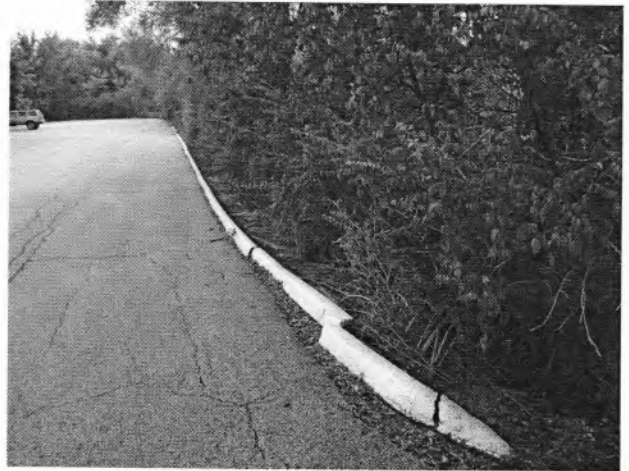
46. Curb line along north side of property
