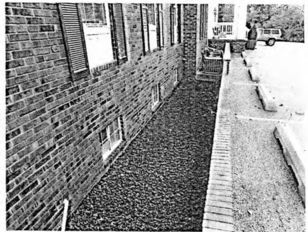
8. Lightwell along north side
