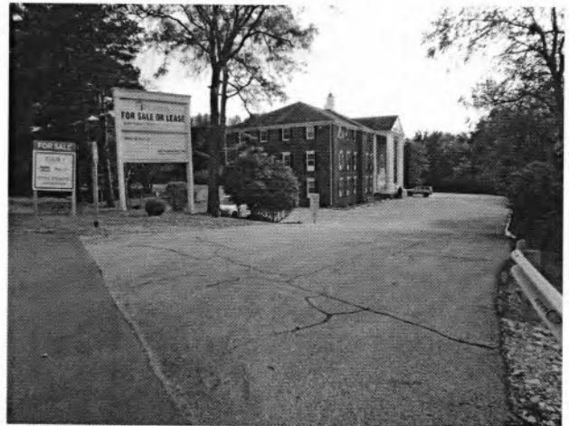
48. Curb cut along main entry drive
