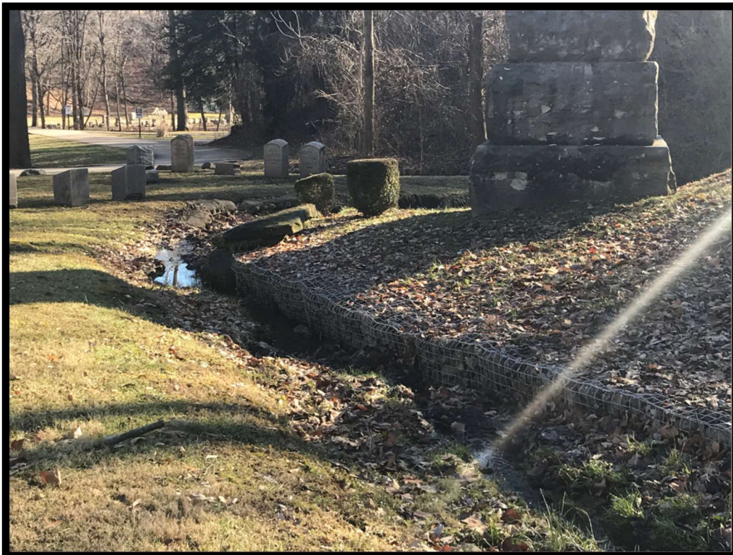
Example of successful channel stabilization project elsewhere in Springdale.
