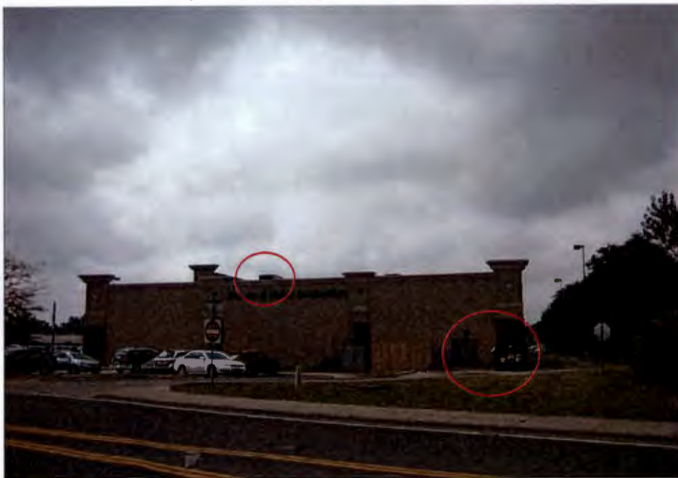
Visible Rooftop HVAC Units & Unscreened Dumpsters
