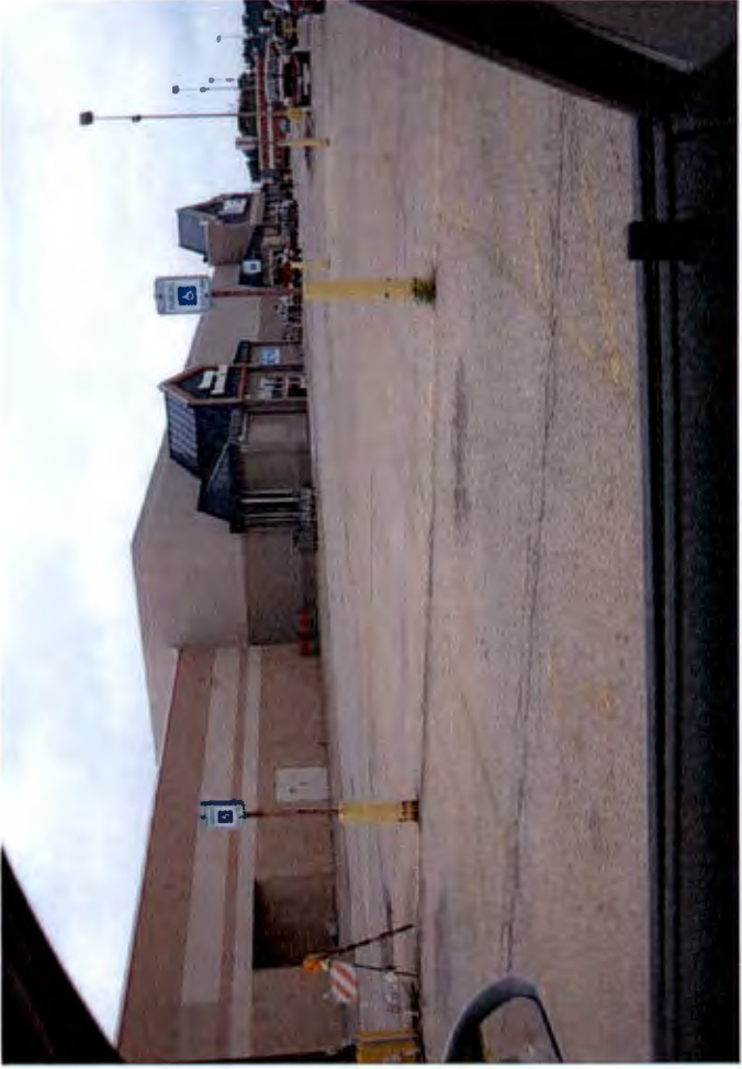
Parking surface in disrepair, improperly signed disabled spaces, fading striping - Old Cub Foods
