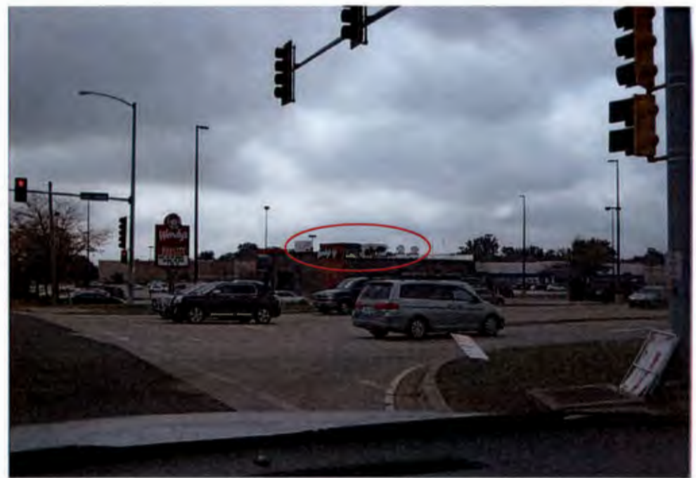
Visible Rooftop HVAC Units
