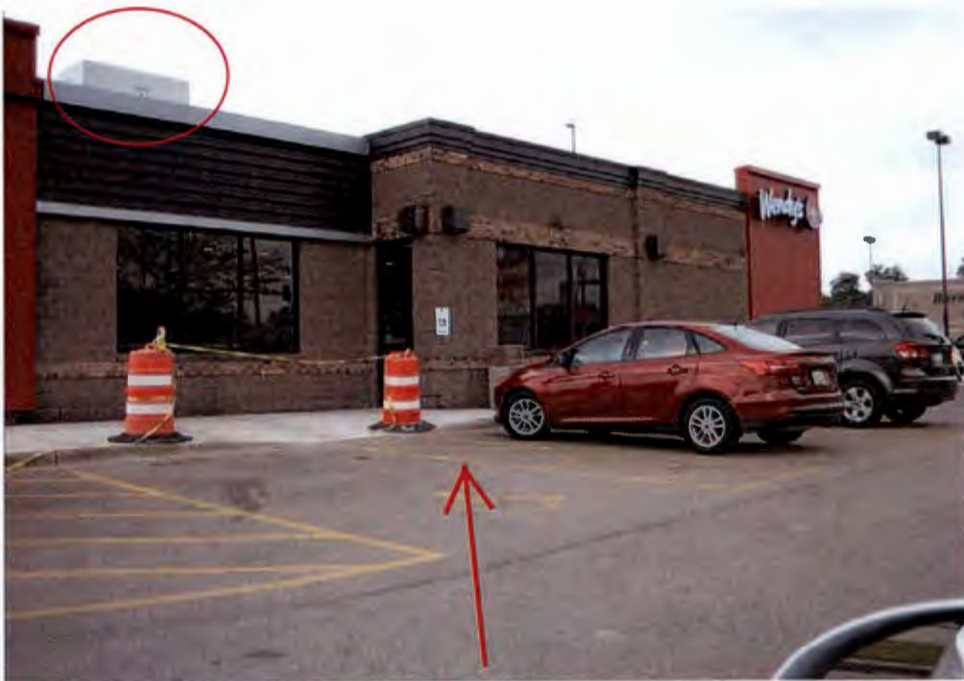
Visible Rooftop HVAC Units & Disabled Spaces not properly signed
