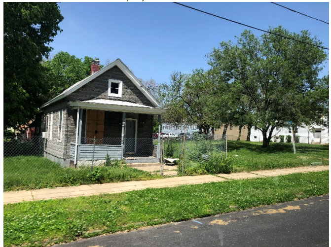
Figure 12 – Vacant lots next to occupied houses highlight the Southside neighborhood's population loss since 1950.
