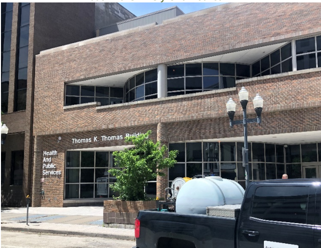
Figure 3 – The Thomas Building is the future site of the Peoria Innovation Hub in Downtown.
