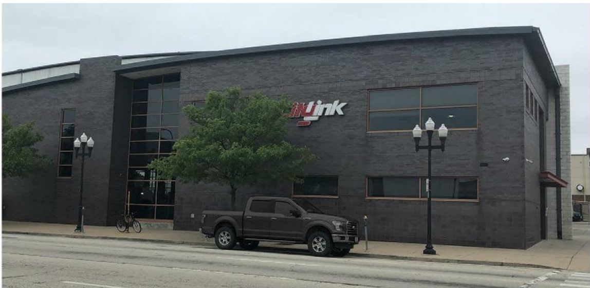
Transit Center – Passenger Transfer
