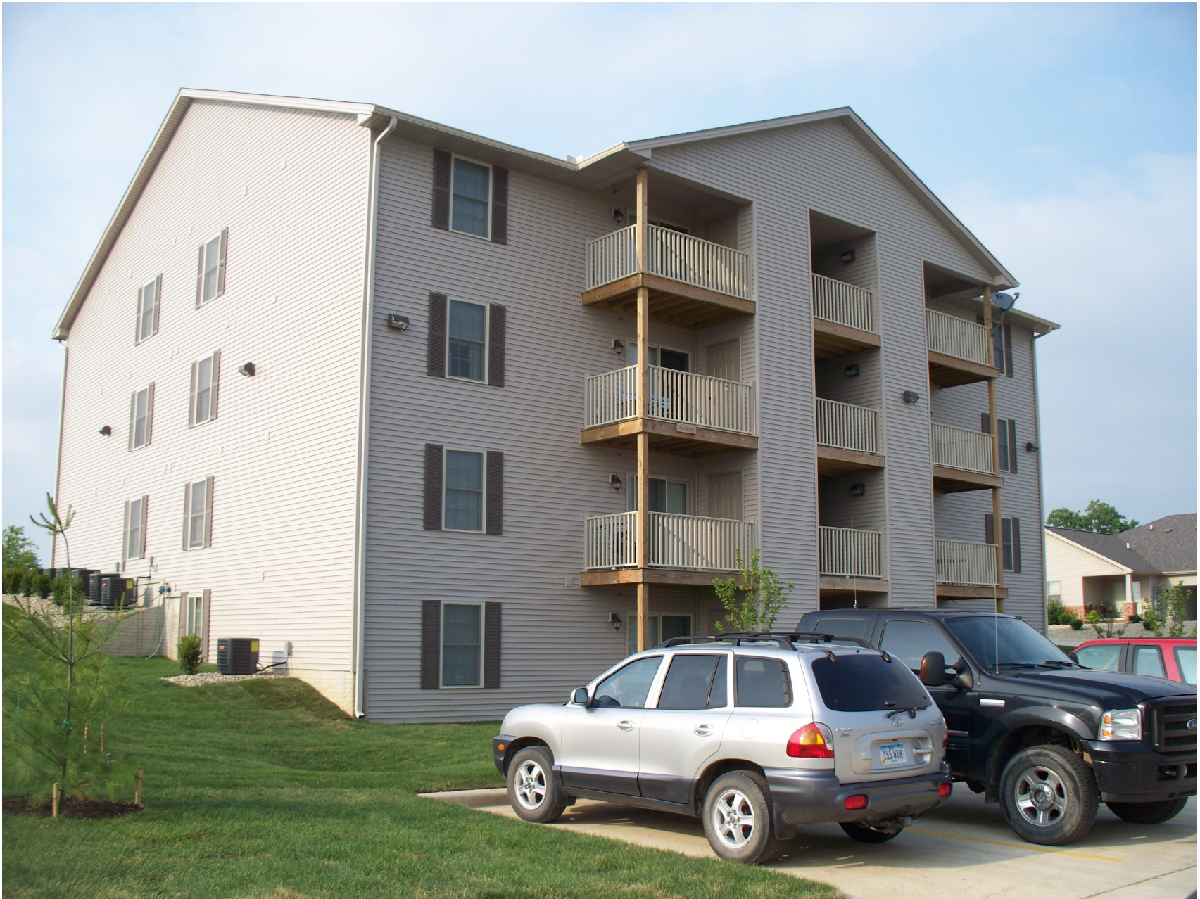
Rear Elevation of Apartment Building Villas at Grand Prairie
