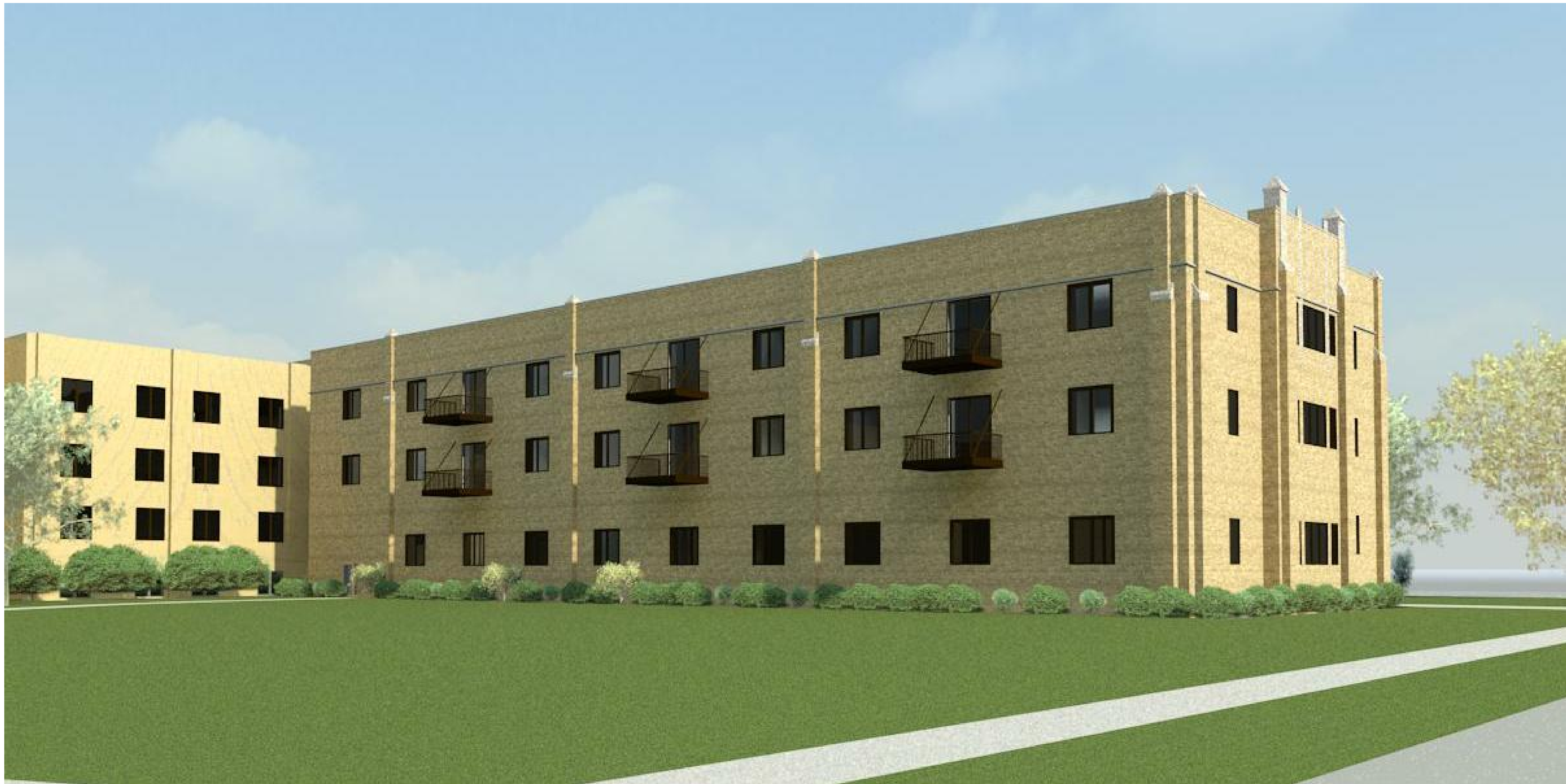
North Addition - View from South
