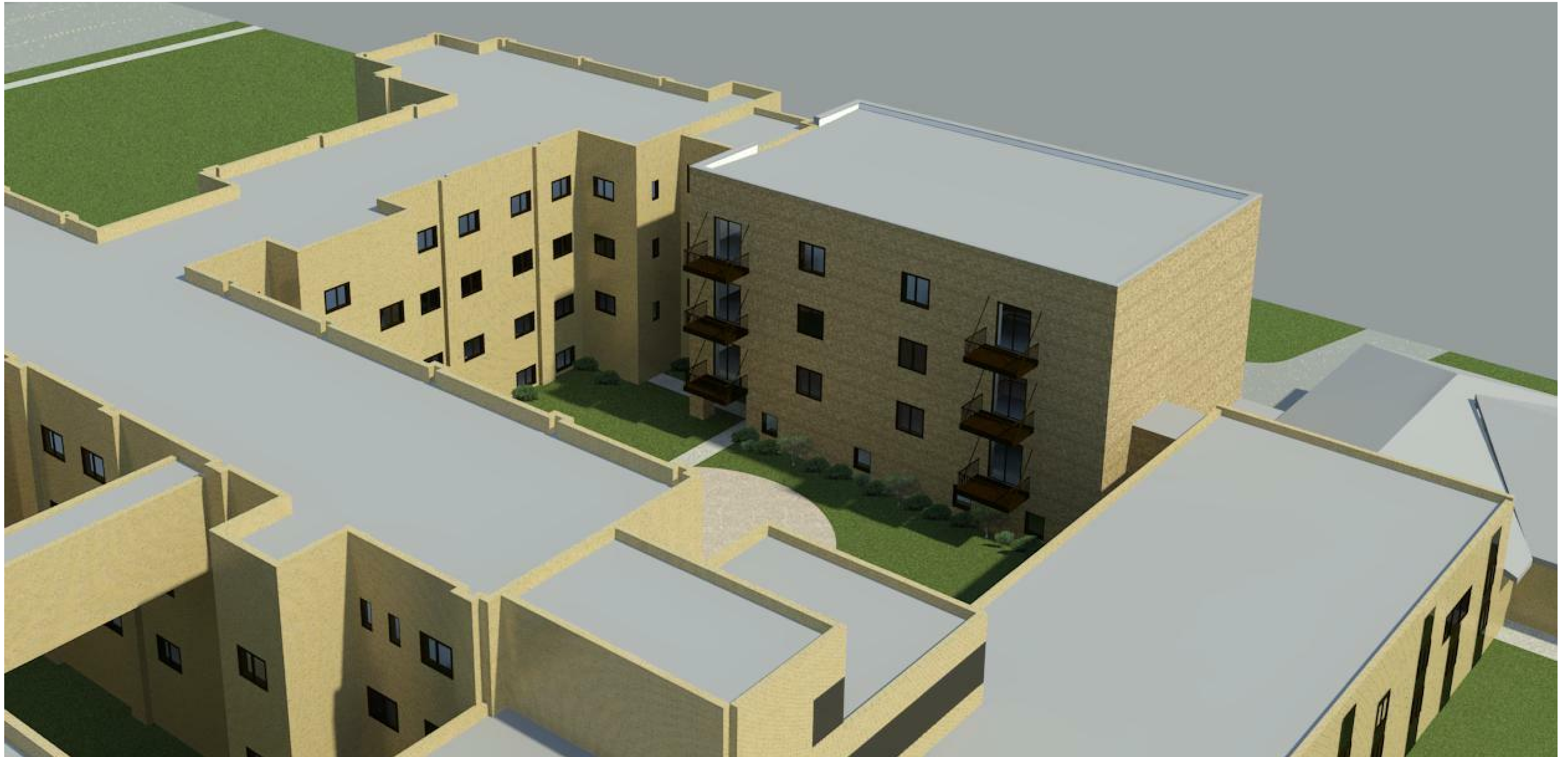
South Addition - Ariel View from North
