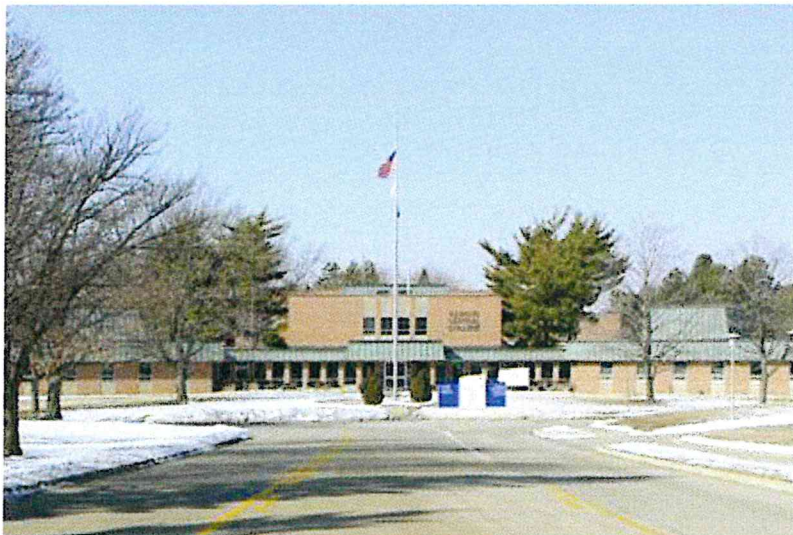
Renovate Arbor Hall - Existing Main Entrance
