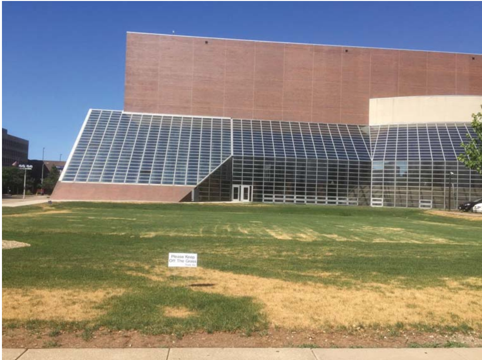
Northeast Elevation (Fulton Street)
