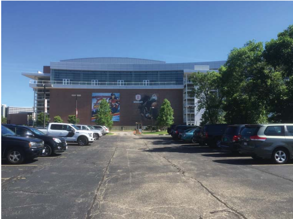
Southwest Elevation (Jefferson Street)
