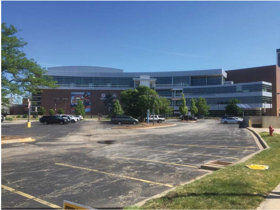
Southwest Elevation (Jefferson Street)
