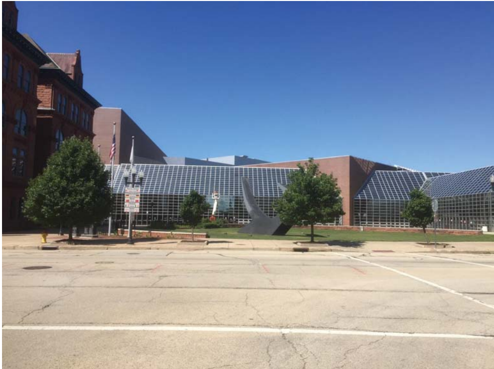
Northeast Elevation (Fulton Street)
