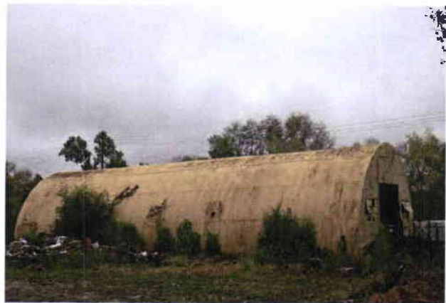
Former quonset hut containing used tires and junkyard salvage
