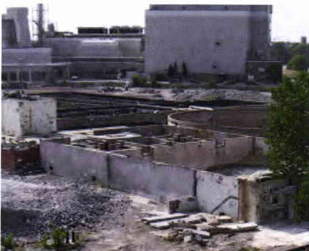
Before: PH Glatfelter Paper Mill Grant Procurement and Implementation, Neenah, WI
