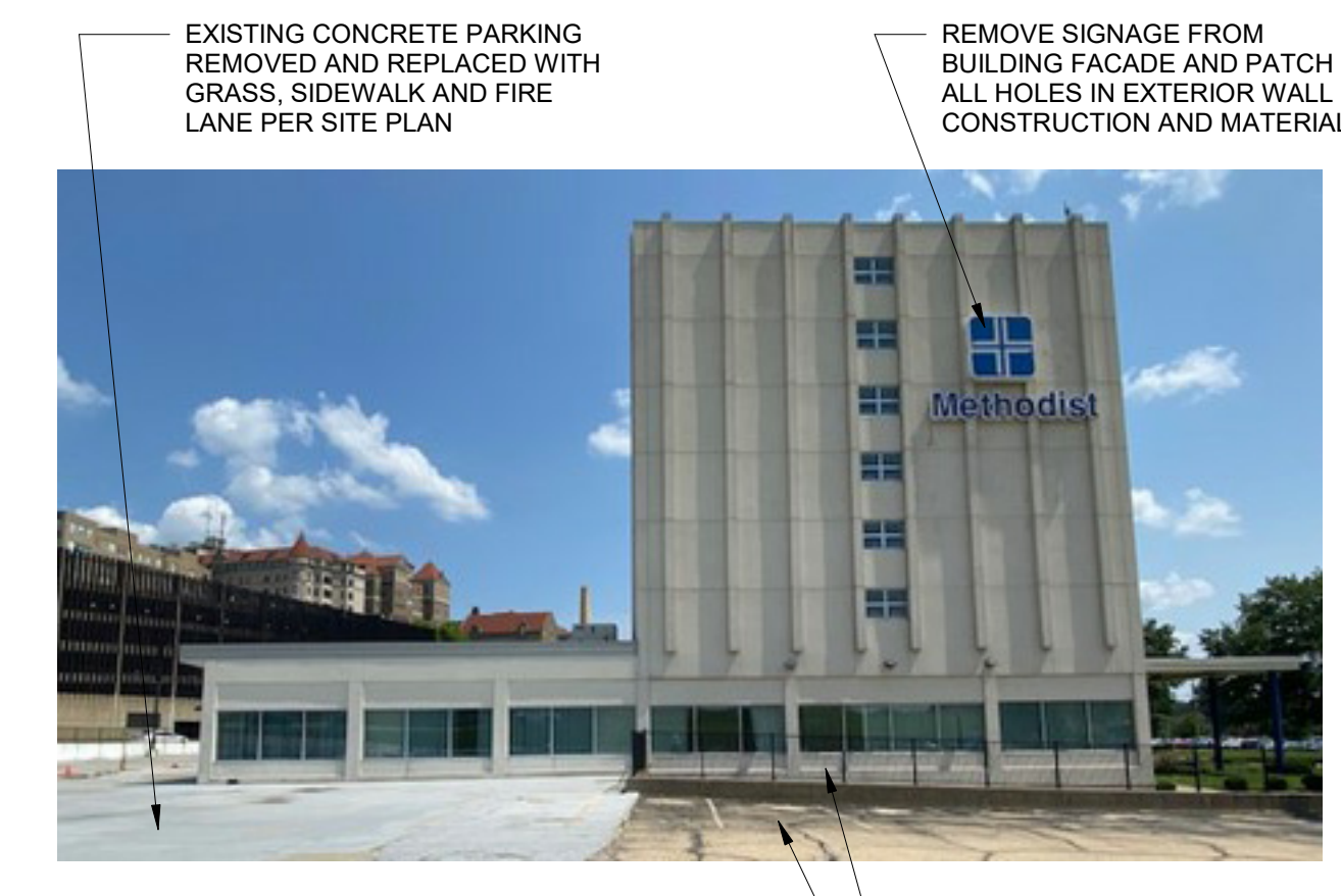
WEST ELEVATION - EXISTING
