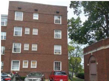
3 EXISTING SOUTH VIEW OF BUILDING SCALE: N.T.S.
