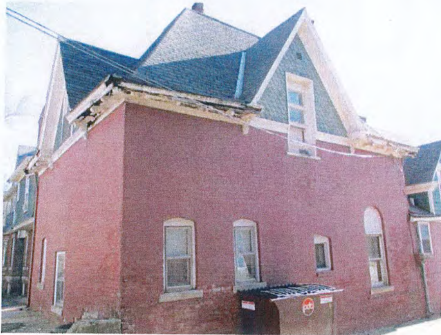
REAR CARRIAGE HOUSE
