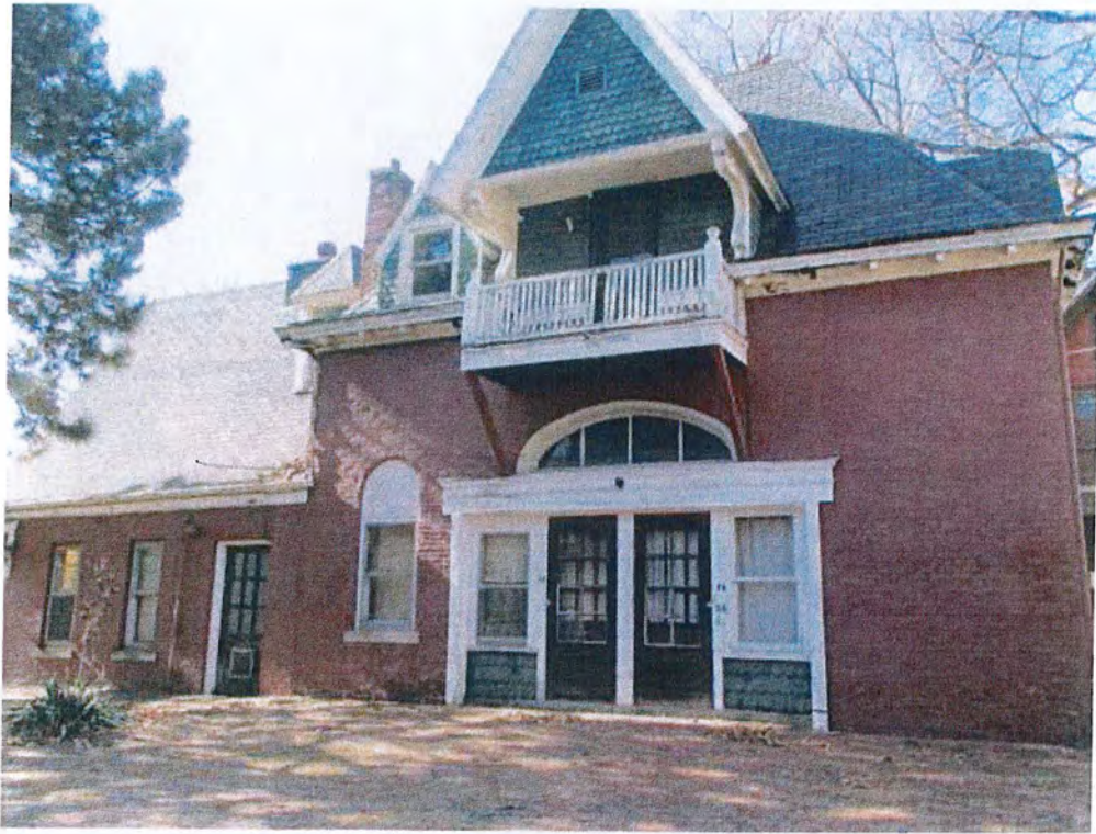
FRONT CARRIAGE HOUSE
