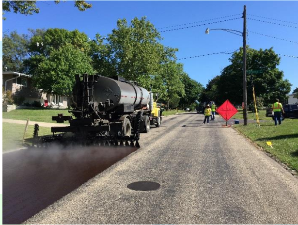
Seal coating oil distributor
