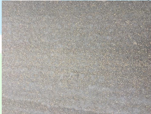
Sealcoating after sweeping
