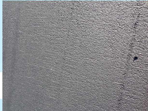
Slurry seal after curing
