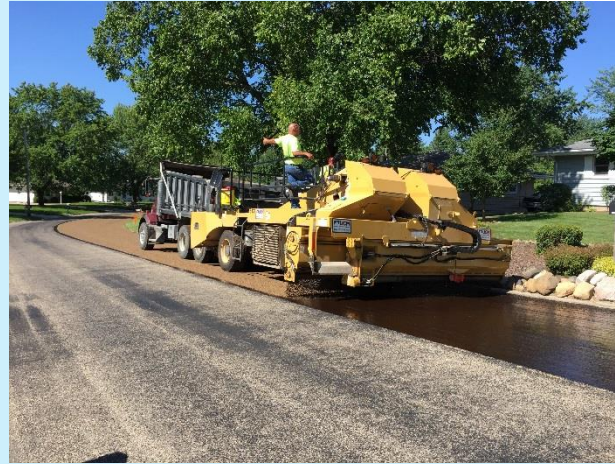
Seal coating rock distributor
