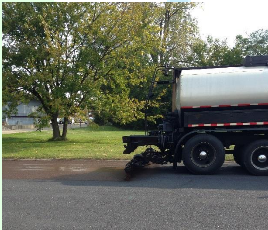
CRF being applied
