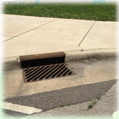
Storm Water Drainage Repair
