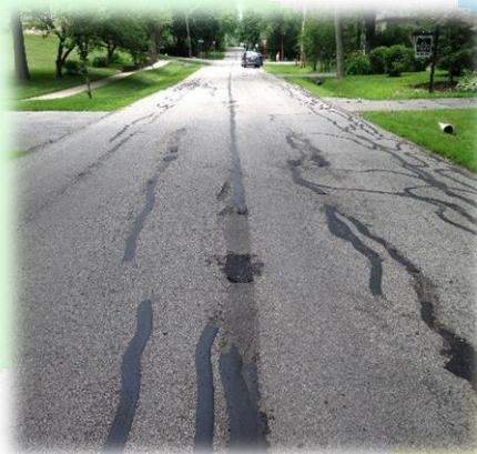
Pavement Preservation Prep
