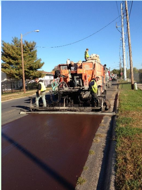
Slurry seal being applied
