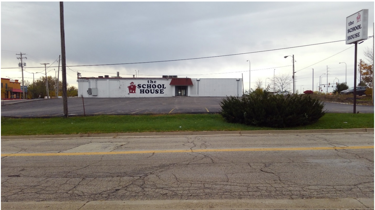
Looking South at North Side of Building
