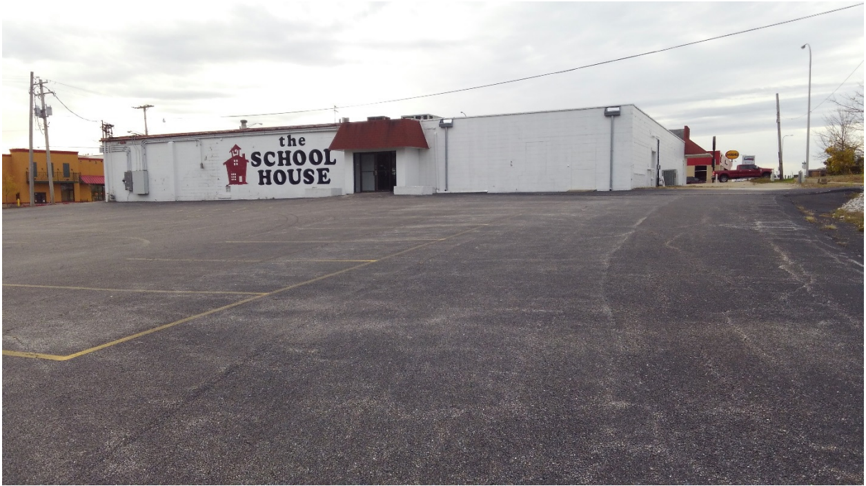
Looking South at North Side of Building
