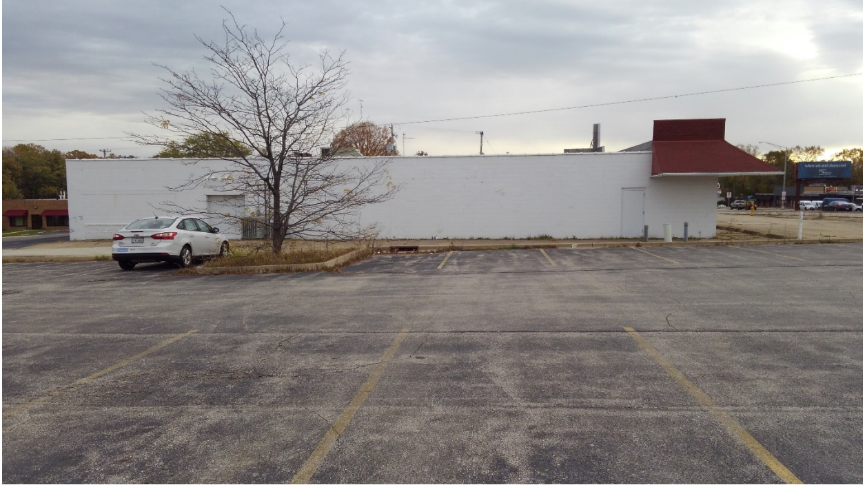
Looking East at West Side of Building
