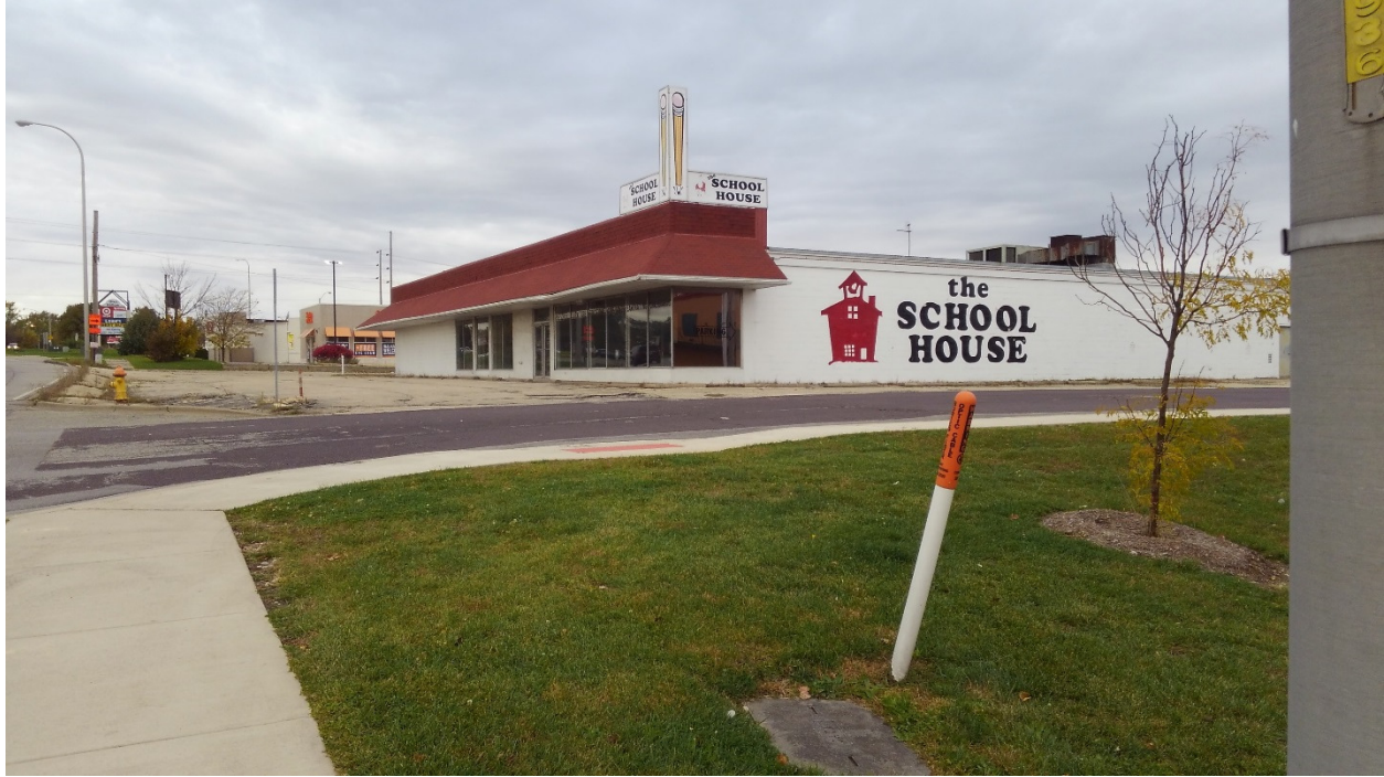
Looking Northwest at Southeast Corner of Building
