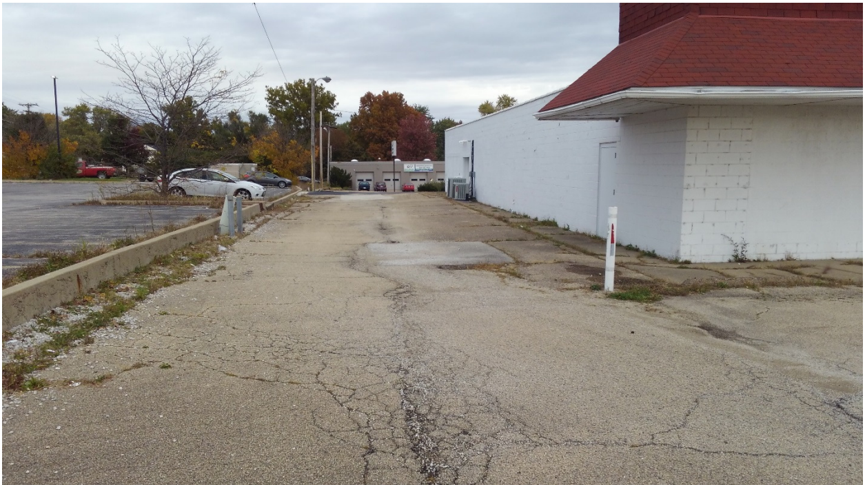
Looking North along West Side of Building
