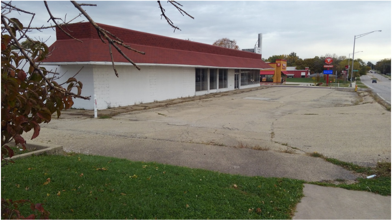
Looking Northeast at South Side of Building
