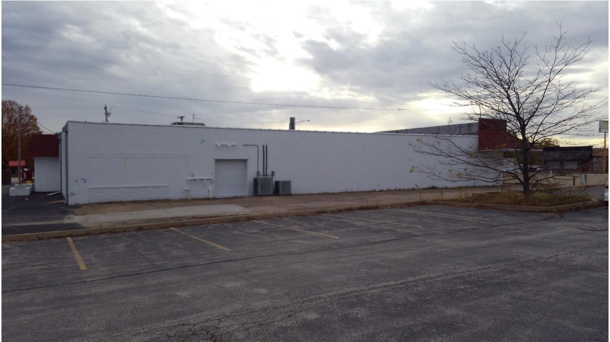
Looking East at West Side of Building
