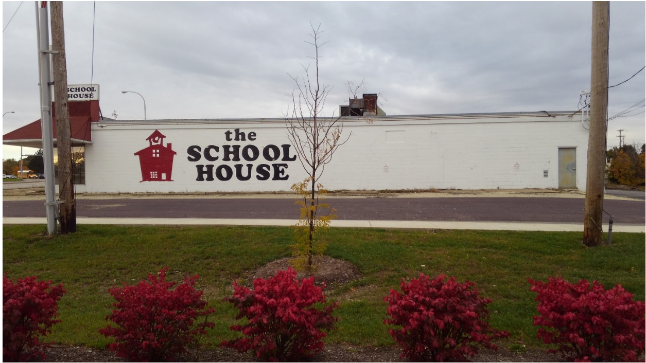
Looking West at East Side of Building
