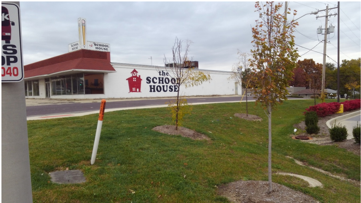
Looking Northwest at East Side of Building
