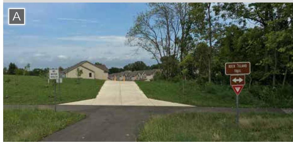
Intersection with Trail by Neighborhood (South of Allen Road)
