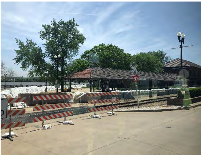
Figure 5 – A railroad station building converted into restaurants is surrounded with sandbags to protect it from river flooding.
