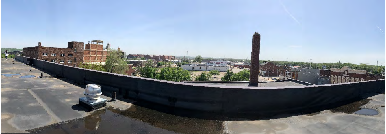
Figure 19 – The 1312 SW Adams Street rooftop overlooks Peoria’s Warehouse District.
