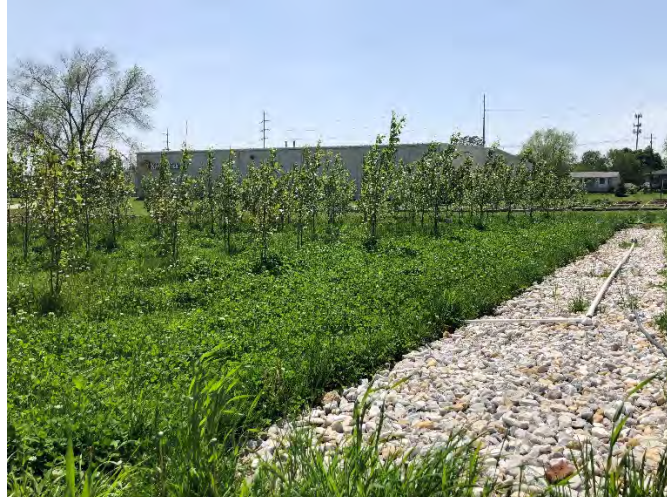
Figure 14 – Trees at the Well Farm absorb stormwater redirected from the City's combined sewer system.
