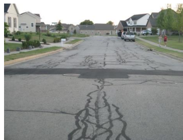
Cracked pavement
