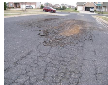
Failed pavement
