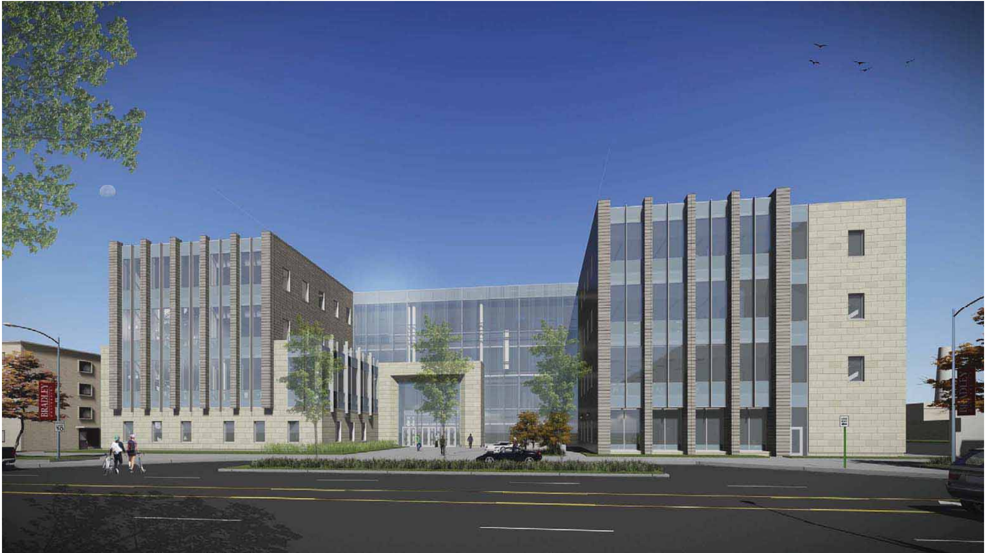
VIEW FROM MAIN STREET LOOKING SOUTH
