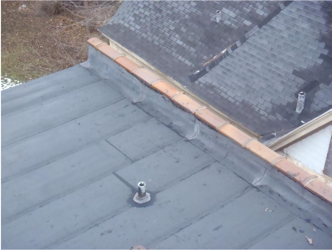
Parapet/flashing repair
