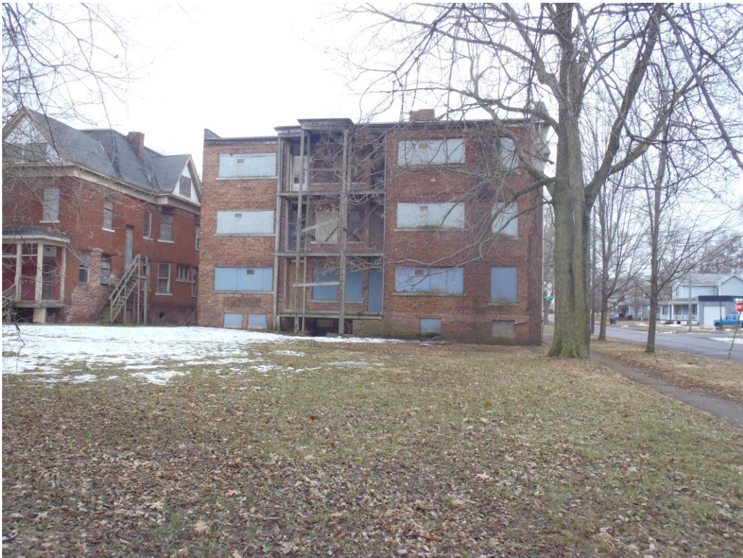
Back of building
