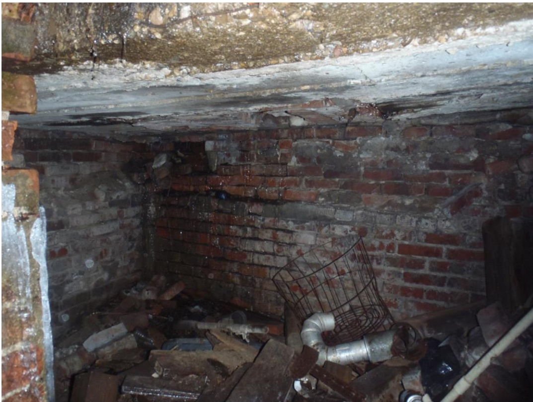
Interior view of exterior wall with falling masonry needing replacement
