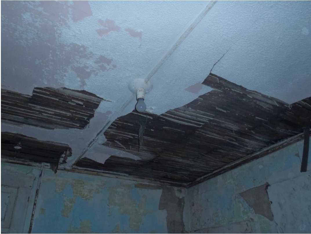
Surface mounted wire ways need to be removed and new wiring installed
