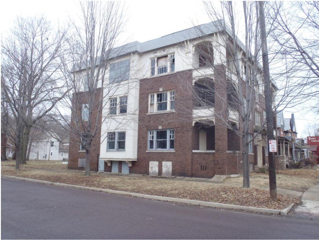
View from corner of Perry Avenue & Wayne Street
