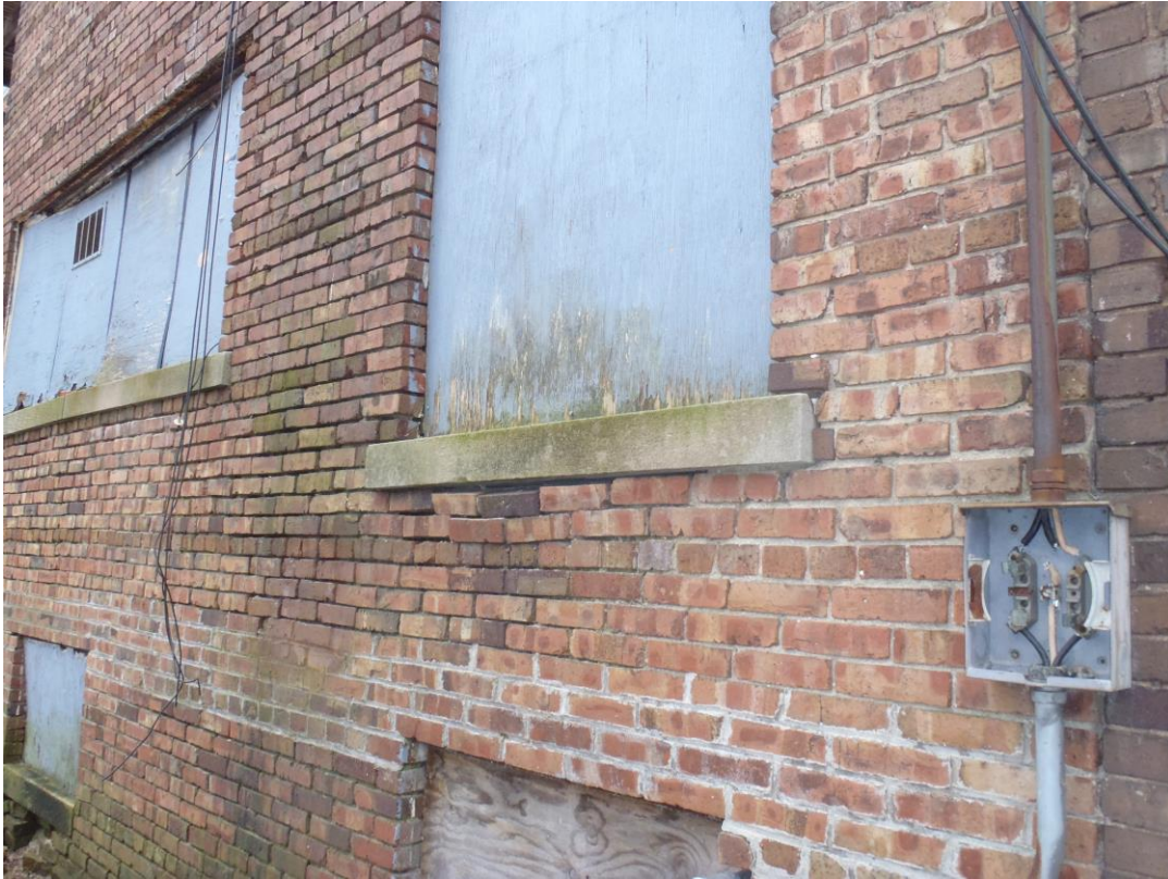
Falling masonry and missing mortar showing extensive need for repair and tuckpointing
