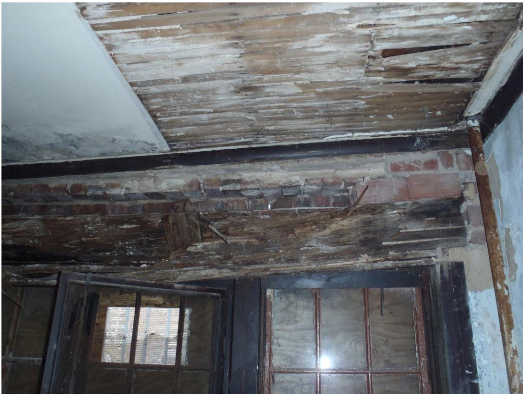
Falling masonry and missing mortar showing extensive need for repair and tuckpointing
