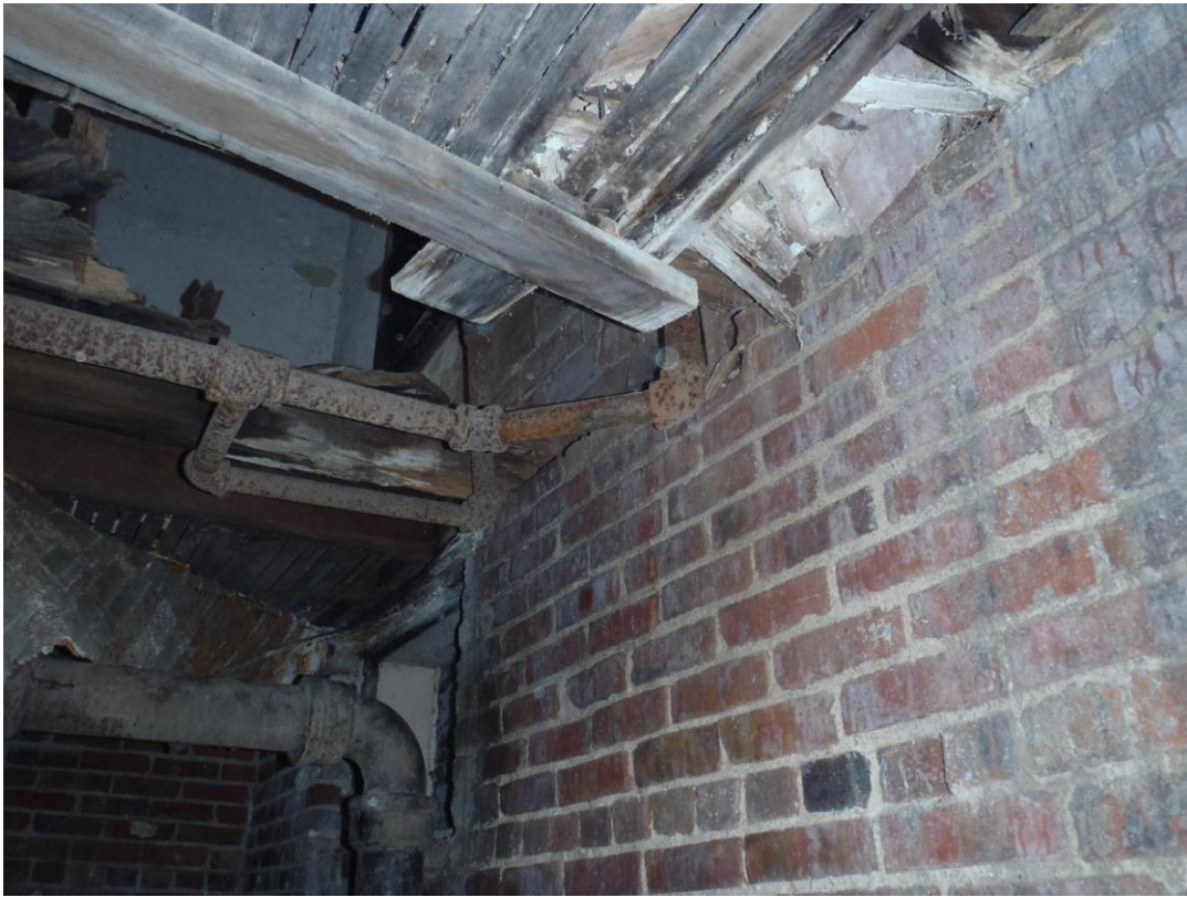
Interior view of exterior wall with falling masonry needing replacement
