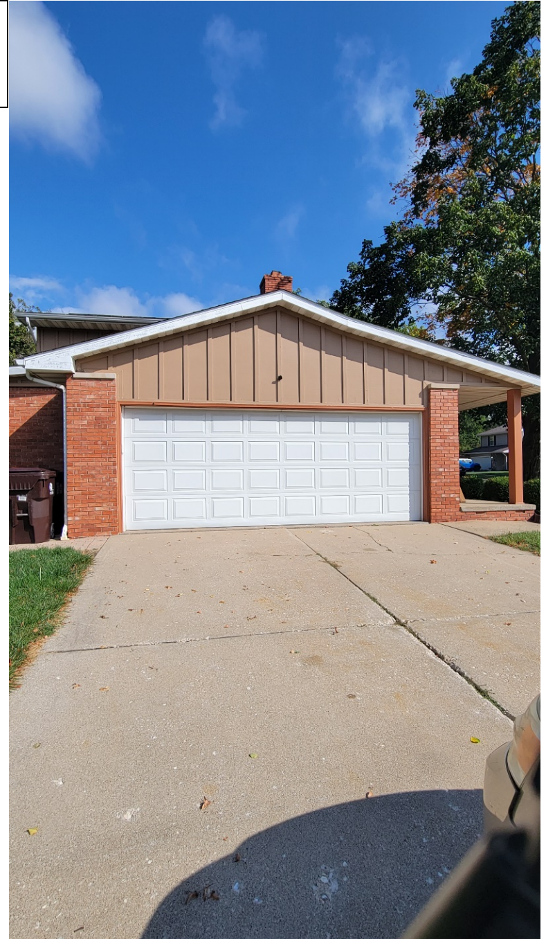
Garage with access from Woodway Dr.
