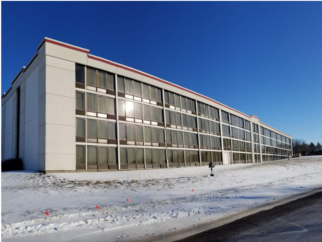
Picture 6 - South-Southwest Elevation
