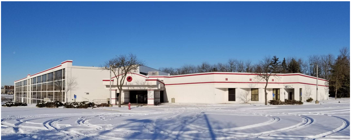
Picture 2 - Southeast Elevation
