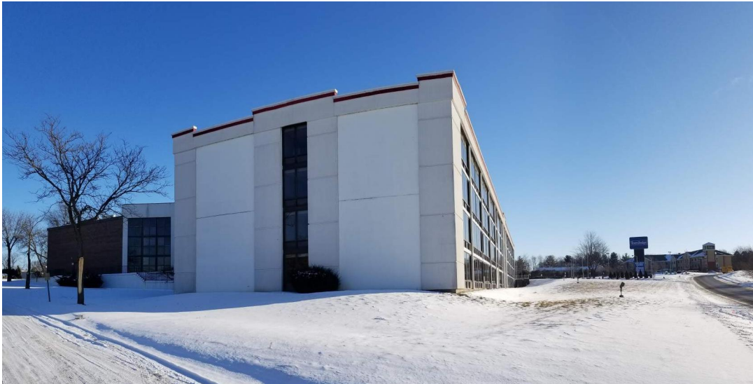
Picture 5 - West-Southwest Elevation
