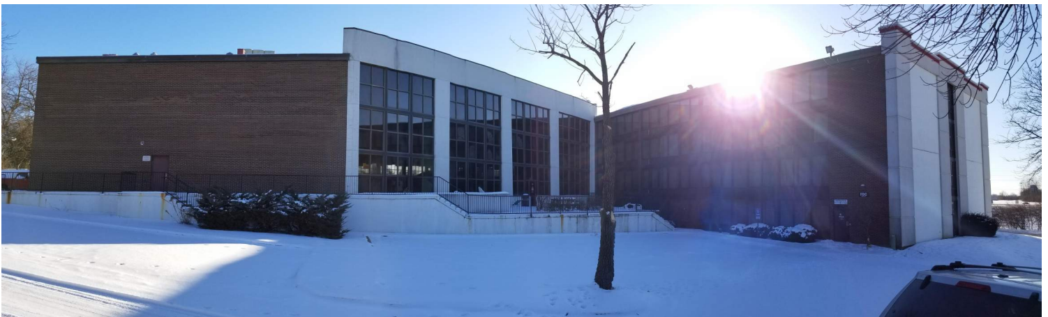
Picture 4 - West Elevation
