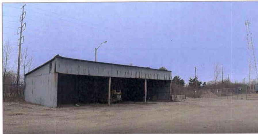
Figure 15. Dilapidated structures were evident on the Keller Station Site, including Buildings 5-6 which were to the right of building shown above and recently demolished (photo 12/7/2021).
