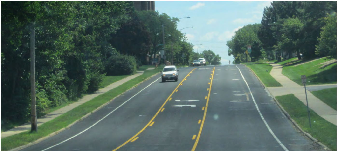
Past planning projects have resulted in travel lane reallocation that one can see in Peoria today.
