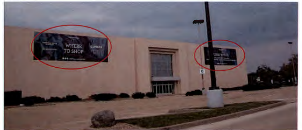
Only one real estate sign allowed per road frontage at max 32 SF, landscaping removed from base of building
