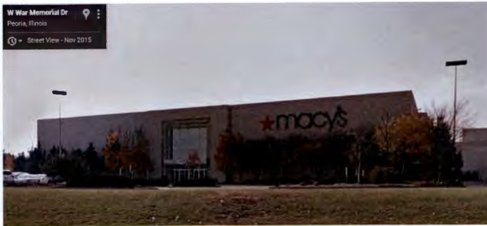
Nov, 2015 Google Street View photo showing previously required landscaping
