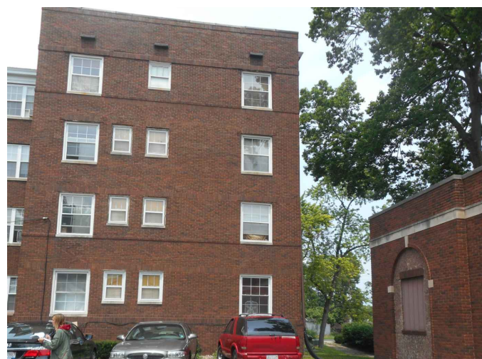
3 EXISTING SOUTH VIEW OF BUILDING SCALE: N.T.S.
