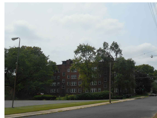
4 EXISTING EAST VIEW OF BUILDING SCALE: N.T.S.
