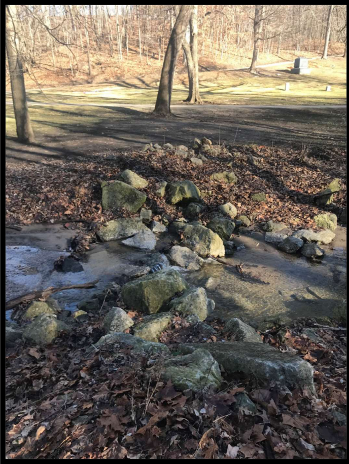
Existing grade control structure at upstream end of project reach.
