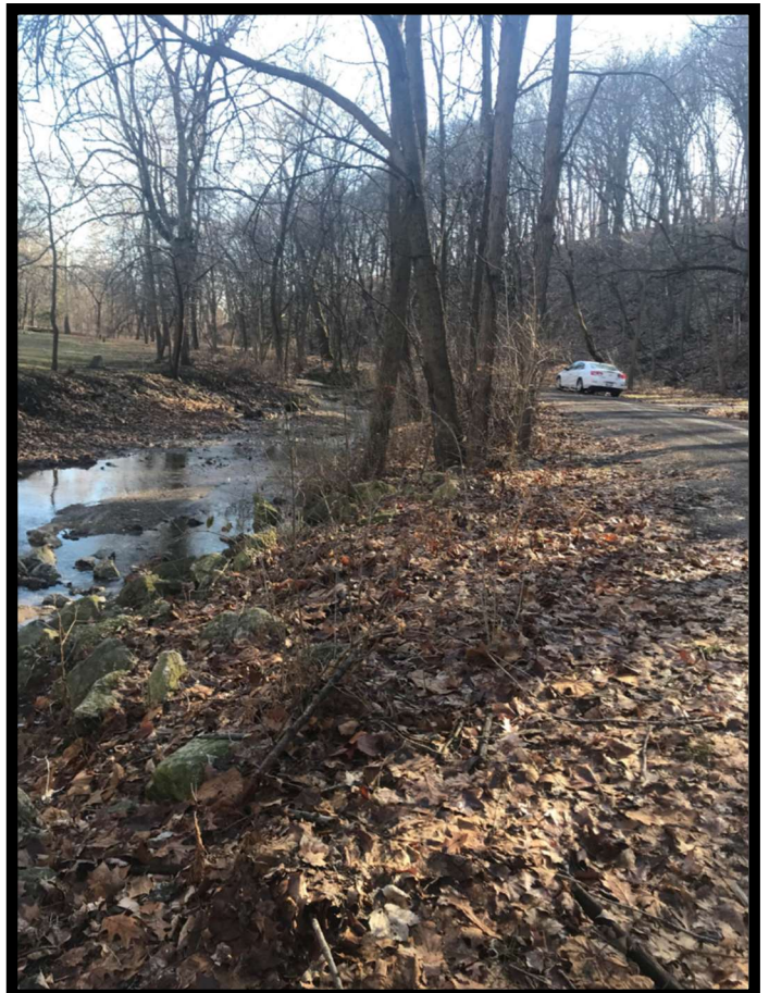
Looking Downstream along project reach from upstream grade control structure
