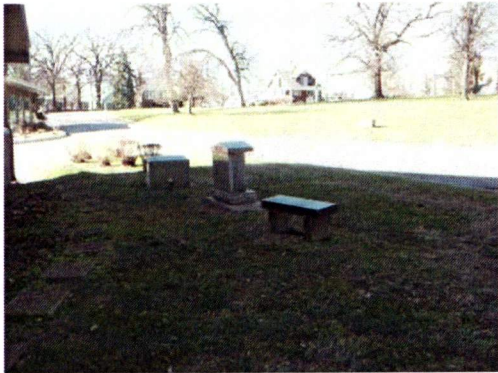
STANDING NORTHEAST OF THE SITE AT THE EXISTING ELECTRIC TRANSFORMER (LOOKING WEST)
