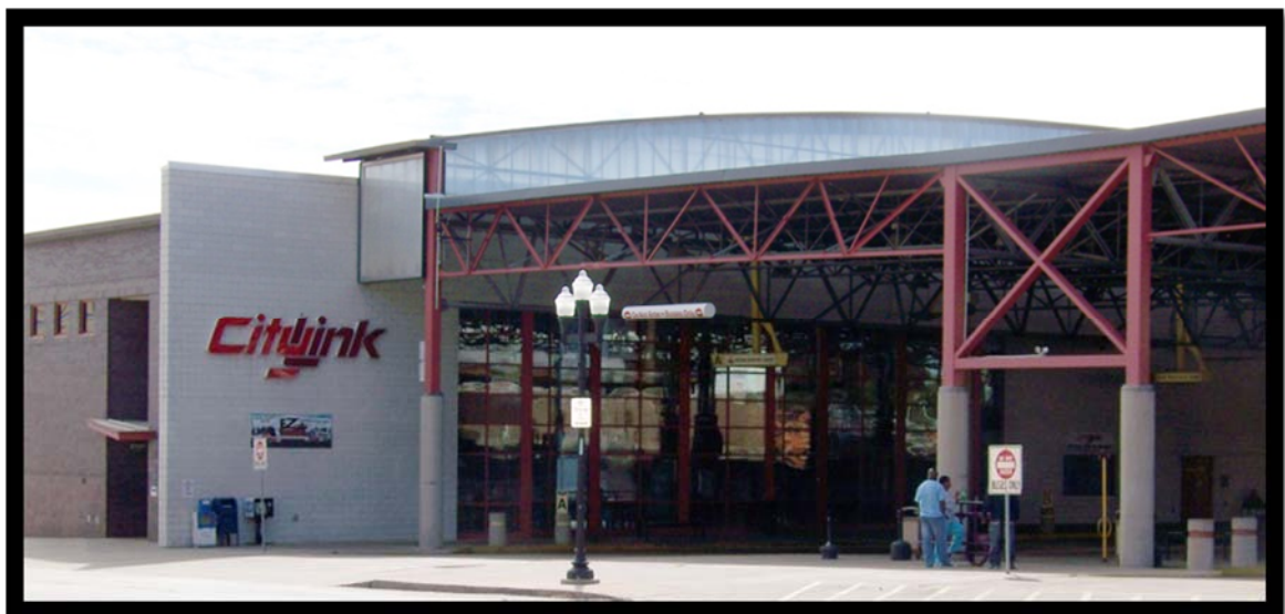
Transit Center – Passenger Transfer
