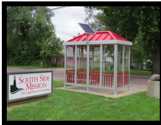
Solar Passenger Shelter (Picture F)
