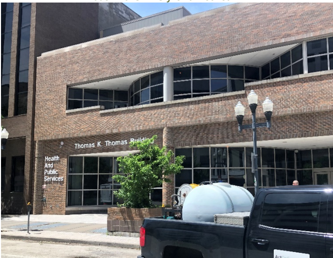
Figure 3 – The Thomas Building is the future site of the Peoria Innovation Hub in Downtown.
