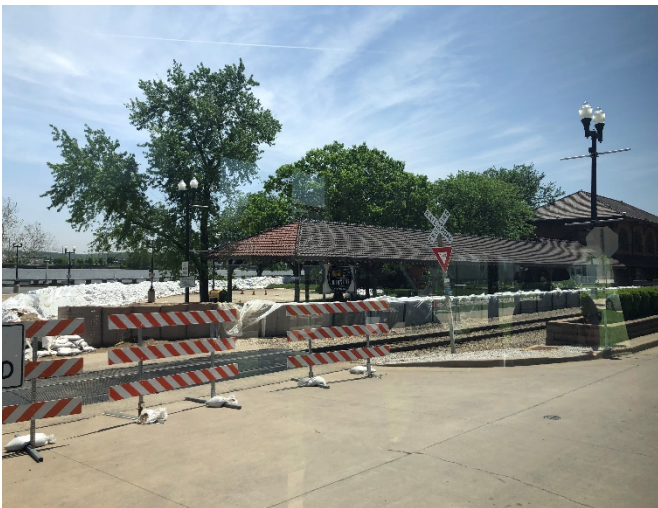
Figure 5 – A railroad station building converted into restaurants is surrounded with sandbags to protect it from river flooding.
