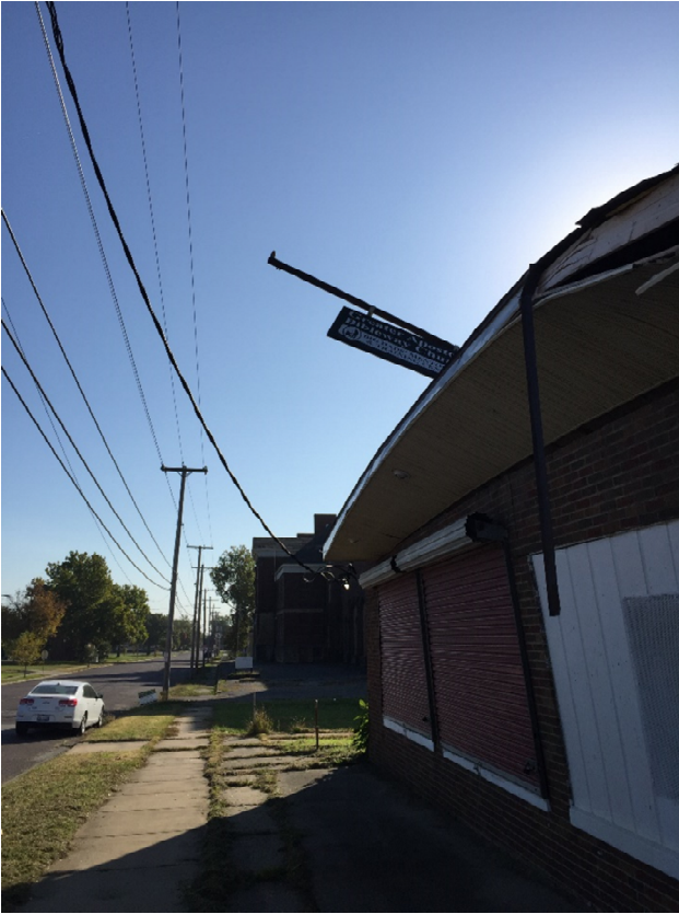
Photo #1 Front of Building
