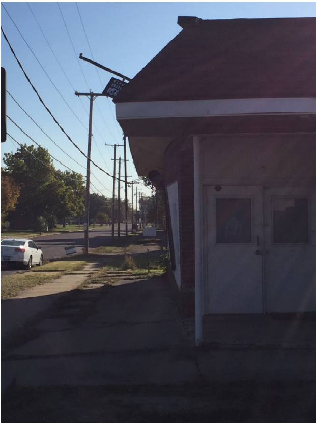
Photo #2 Front of Building
