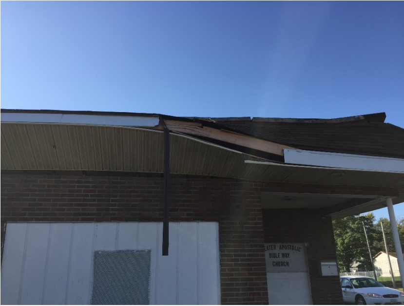
Photo #3 Front of building, awning rotation
