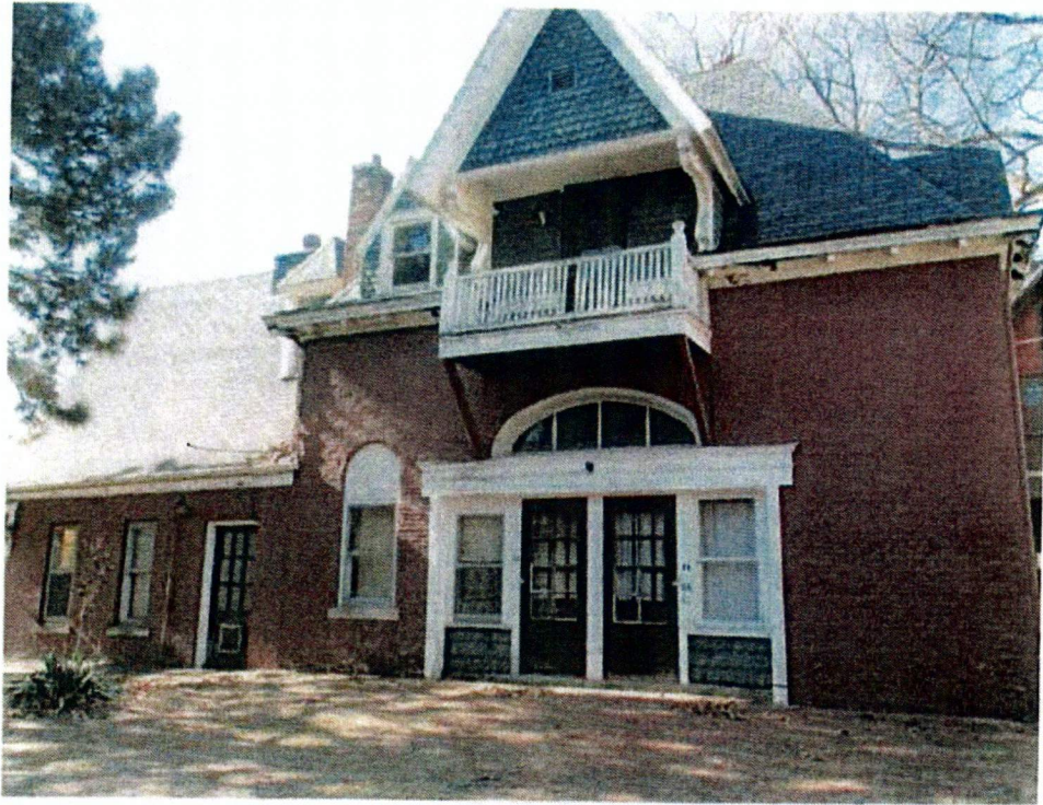
FRONT CARRIAGE HOUSE
