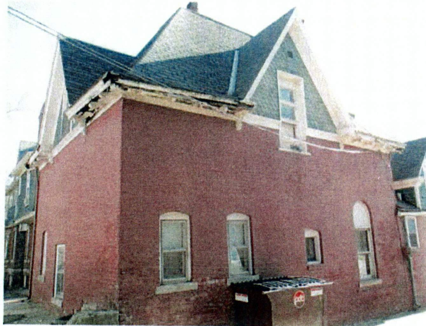
REAR CARRIAGE HOUSE
