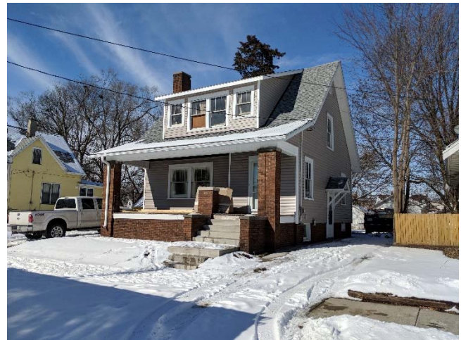
Exterior – Current progress
