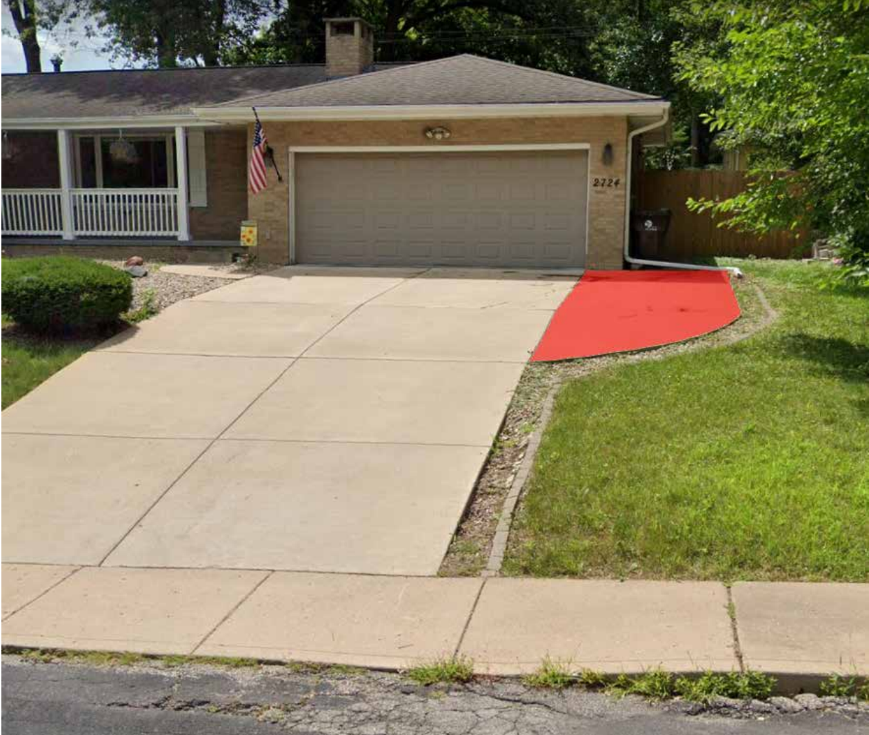
Non-Conforming Driveway Extension
