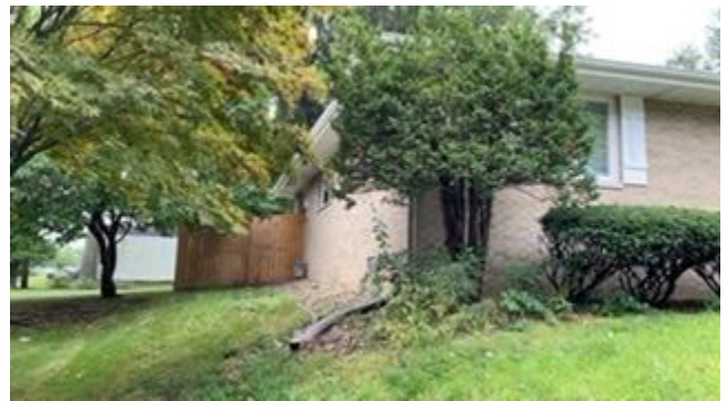
East Face of House (Looking South)
