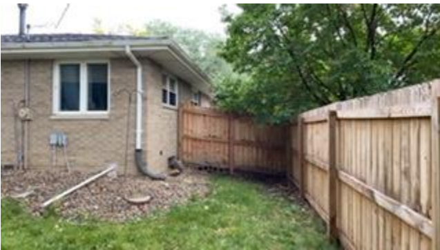
East Face of House (Looking North)
