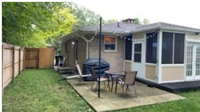
West Face of House
