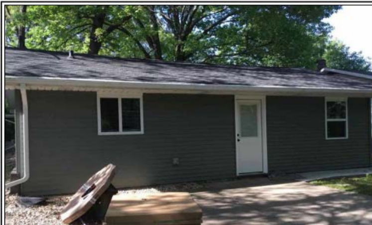
REAR OF SUBJECT PROPERTY
