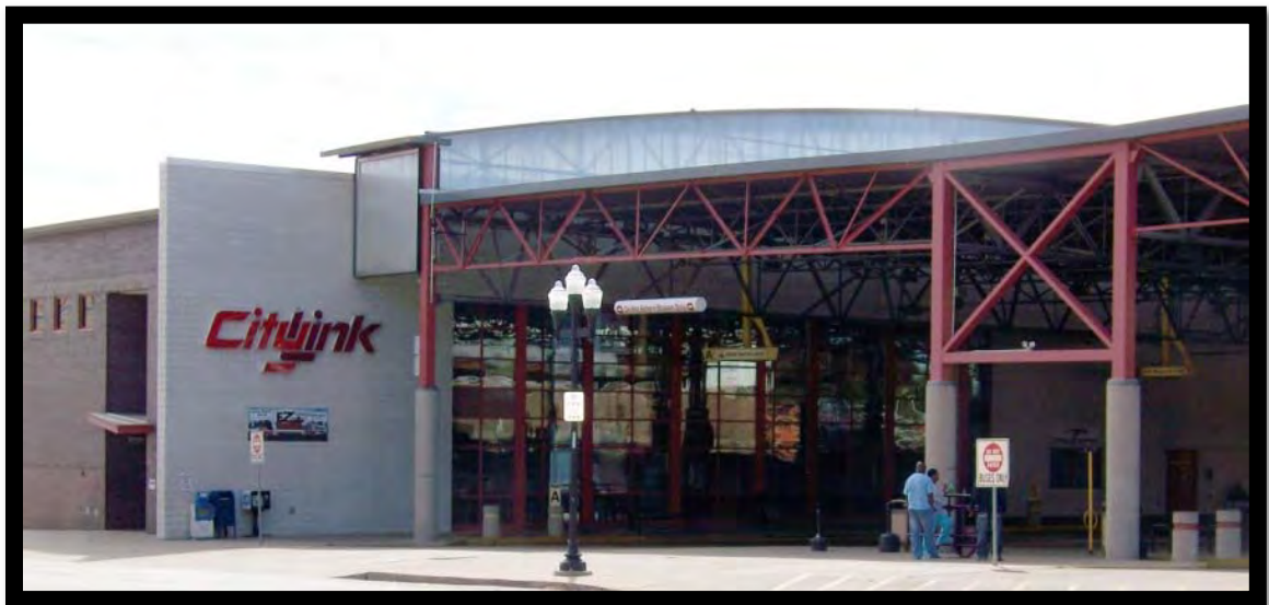
Transit Center – Passenger Transfer
