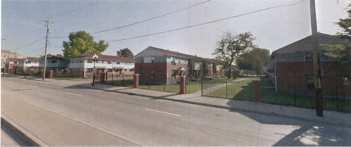
Street view of project site from Eaton St.
