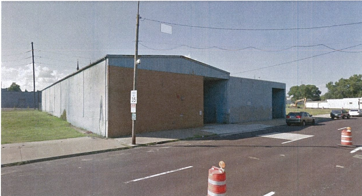
Building north of the project site
